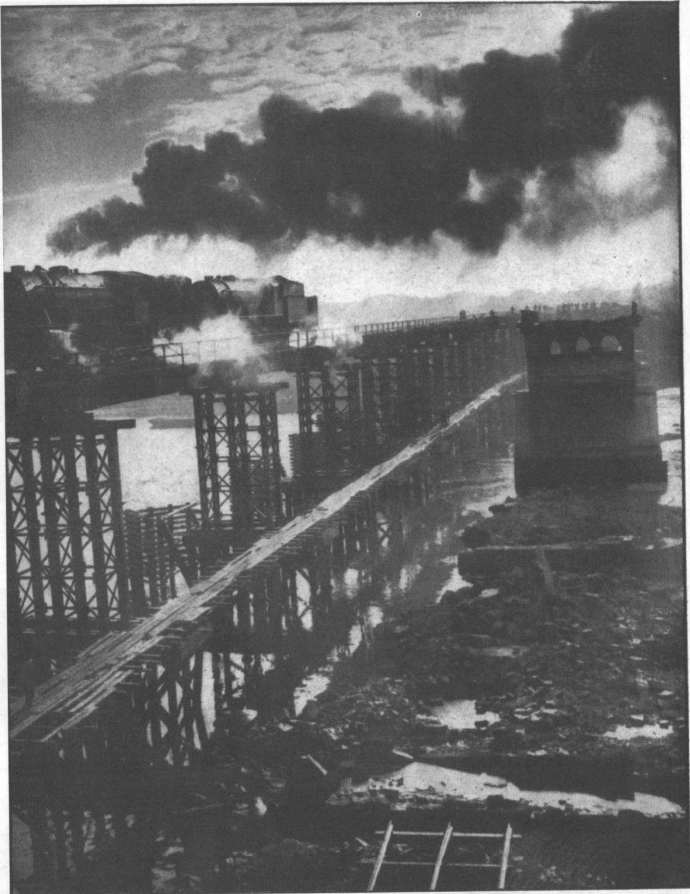
PONT DE LA VENDÉE, SPANNING THE LOIRE, at Nantes, France, was opened to traffic in December 1945, after its strength and stability had been tested by locomotives, weighing 250 tons, which are seen nearing the completion of their run. A temporary structure, 700 yards long, this bridge replaces the original whose ruins are to the right. The construction, commenced in April 1945, entailed the use of 1,600 tons of steel. During the War nearly 3,000 bridges were destroyed in France by the retreating Germans and by Allied bombing.
