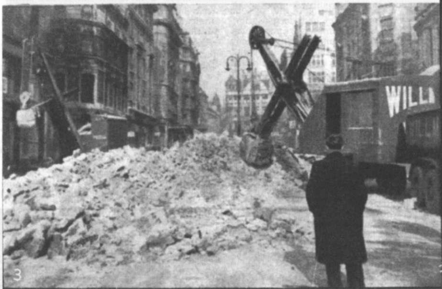
AIR-RAID SHELTER DEMOLITION in Lower Regent Street, London, was conducted at high speed, mechanical navvies working throughout the night (1), some pounding the structures to rubble with solid steel balls (2), others scooping the masonry into lorries with great clawed shovels (3).
