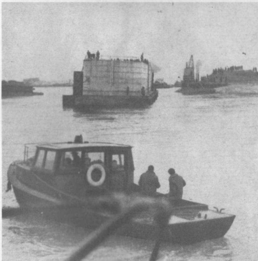
TO SEAL THE BREACHES AND DRAIN THE WATER from flooded Walcheren Island, Dutch workmen have been toiling day and night. One of the concrete caissons of Mulberry Harbour (used for the landings on the Normandy beach-head) is being positioned in the fourth and final gap in the sea-wall.
