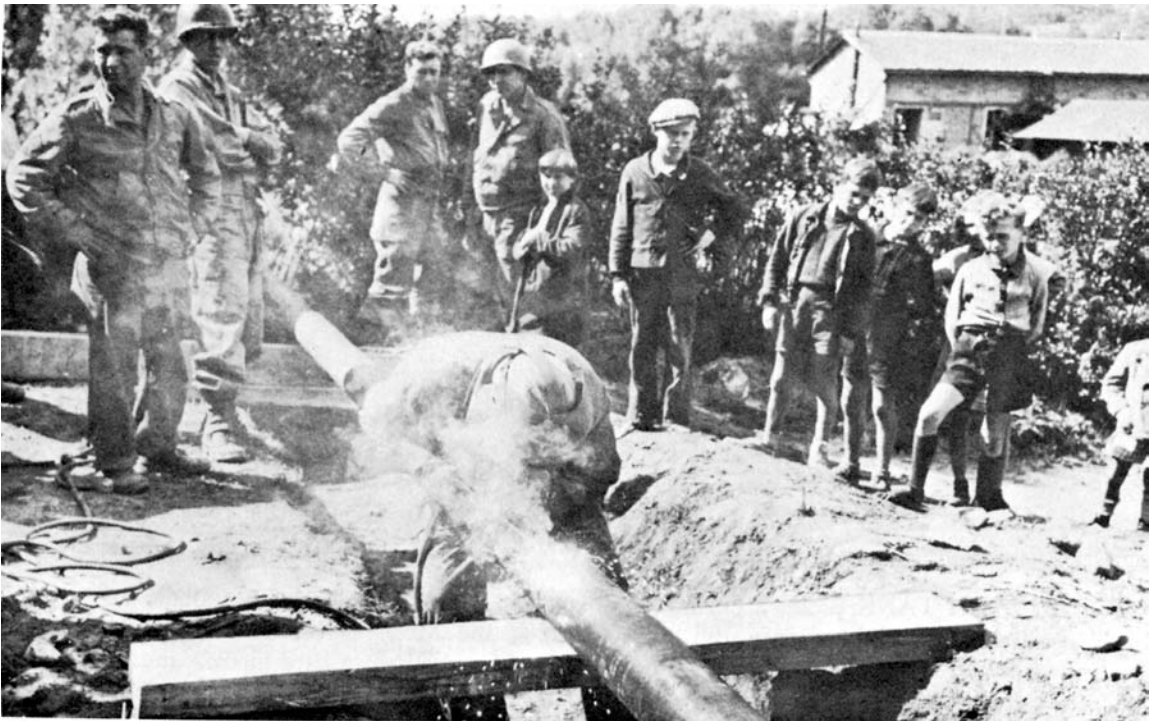
ENGINEERS LAYING A GASOLINE PIPELINE in France. In an effort to transport fuel to the front-line units of the Allies, three fuel pipelines were laid across France. This also relieved the road traffic which became more and more congested as the number of Allied troops in France increased.
