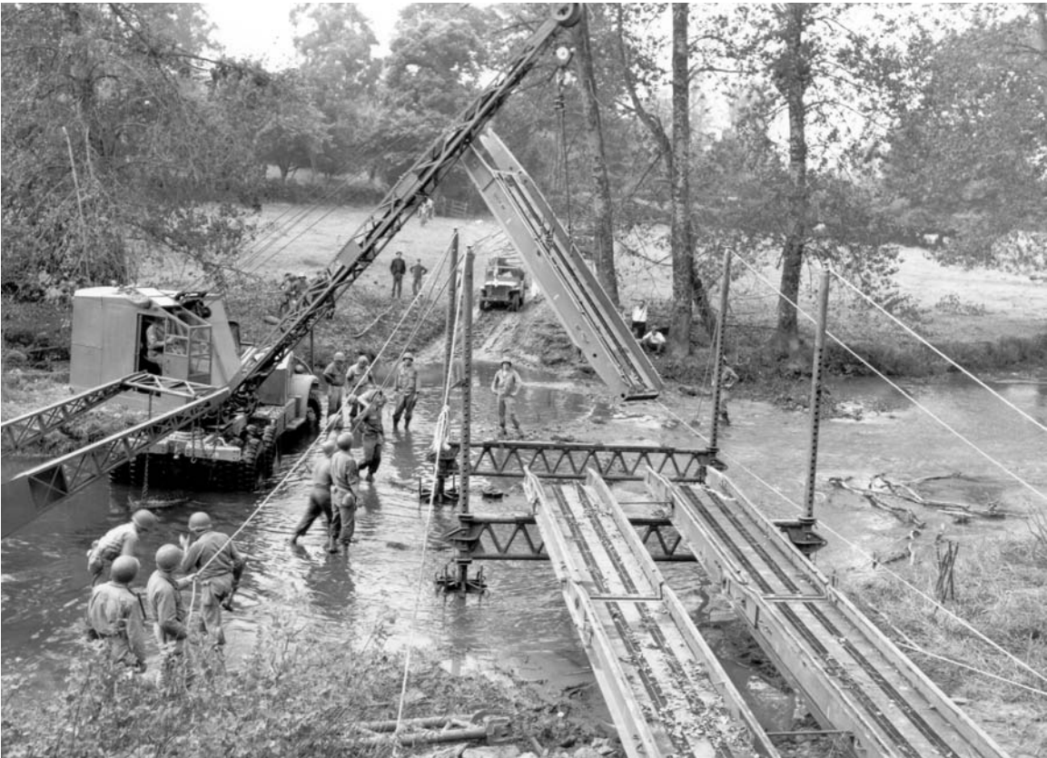
A BULLDOZER (tractor, earth moving crawler, diesel) pulling a jeep from a crater (top). Engineers using a truck-mounted revolving crane swing a section of a tread-way bridge into place over the Vire River near Pontfarcy (bottom).
