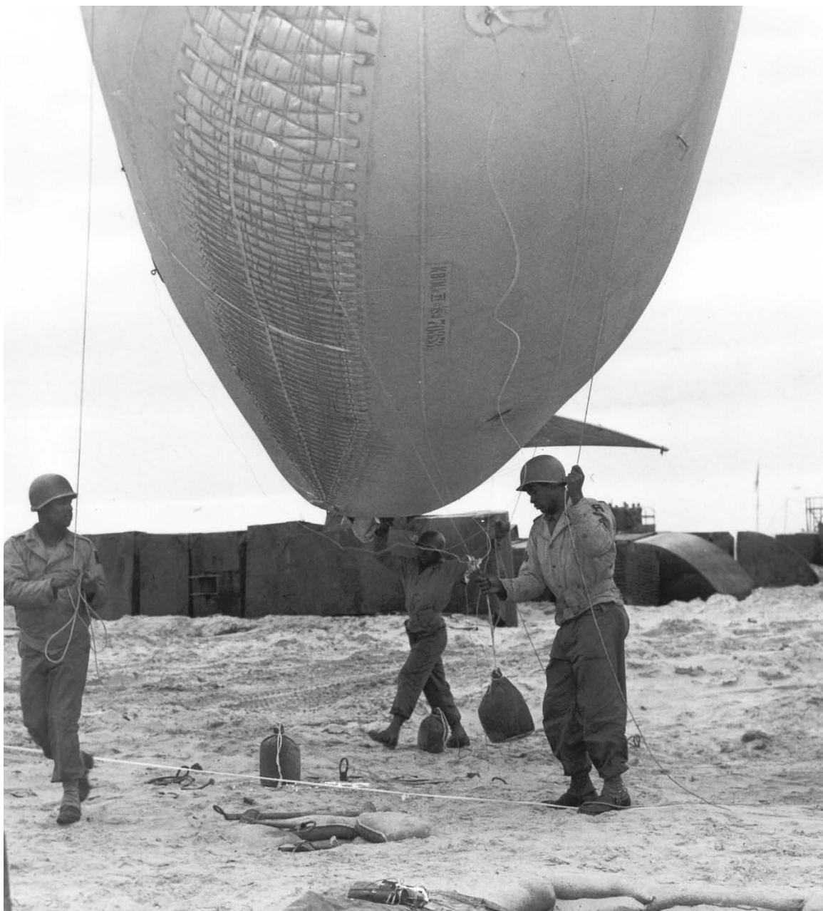
ENLISTED MEN PREPARE TO LAUNCH A BARRAGE BALLOON over one of the beaches in Normandy. Balloons were attached to cables and by means of winches could be raised or lowered to the desired altitude. These balloons were used to protect ships and beach installations from low-flying enemy aircraft. When the balloons were in position the enemy would not fly low over the beaches for fear of running into the cables which kept the balloons in place.
