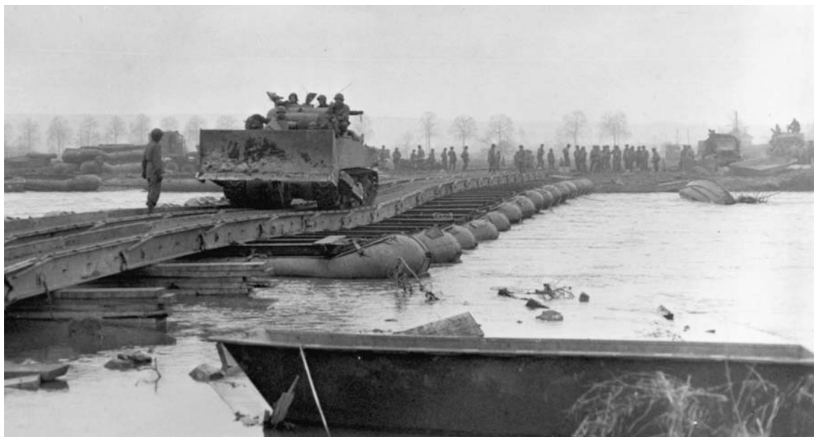
ROER RIVER TREADWAY PONTON BRIDGES. Early on the morning of 23 February the Ninth Army jumped off after a heavy artillery preparation. Covering the right flank was a corps of the First Army. Because the enemy was surprised by this attack only moderate opposition was encountered and by the end of the first day bridgeheads two to four miles deep were held, infantry troops were east of the Roer River, and seven bridges were being completed under a heavy screen of smoke.
