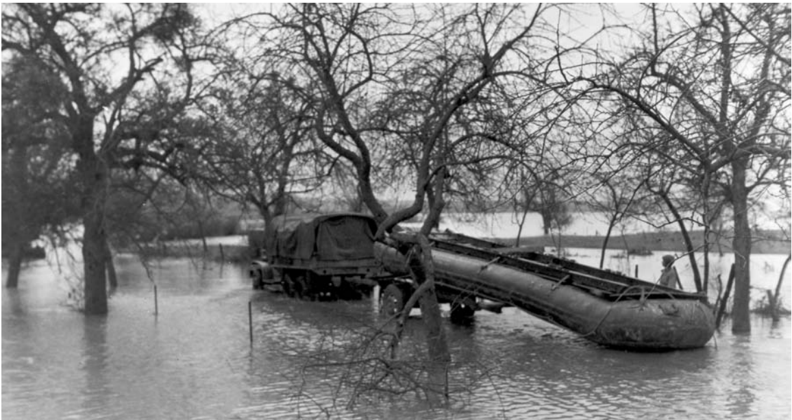
ENGINEERS HAULING BRIDGING EQUIPMENT in flooded areas of the Moselle River. The flooded rivers and smaller streams made the task of bridging extremely difficult during this period of the fighting along the German frontier since, in addition to the wider than normal spans necessary to cross the rivers, the weather was cold and rainy, adding to the hardships of those employed in the task.
