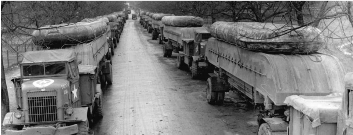
PONTON BOATS AND FLOATS being moved to the Rhine in the Remagen area (top). Treadway bridge across the Rhine near Remagen (bottom). During the period 11–16 March the bridgehead was expanded north and south and all attacks gained ground despite the arrival of enemy reinforcements. Treadway and heavy pontoon bridges were built across the river. As the Rhineland Campaign came to an end, six divisions were east of the Rhine and six more were ready to cross in the First Army zone.
