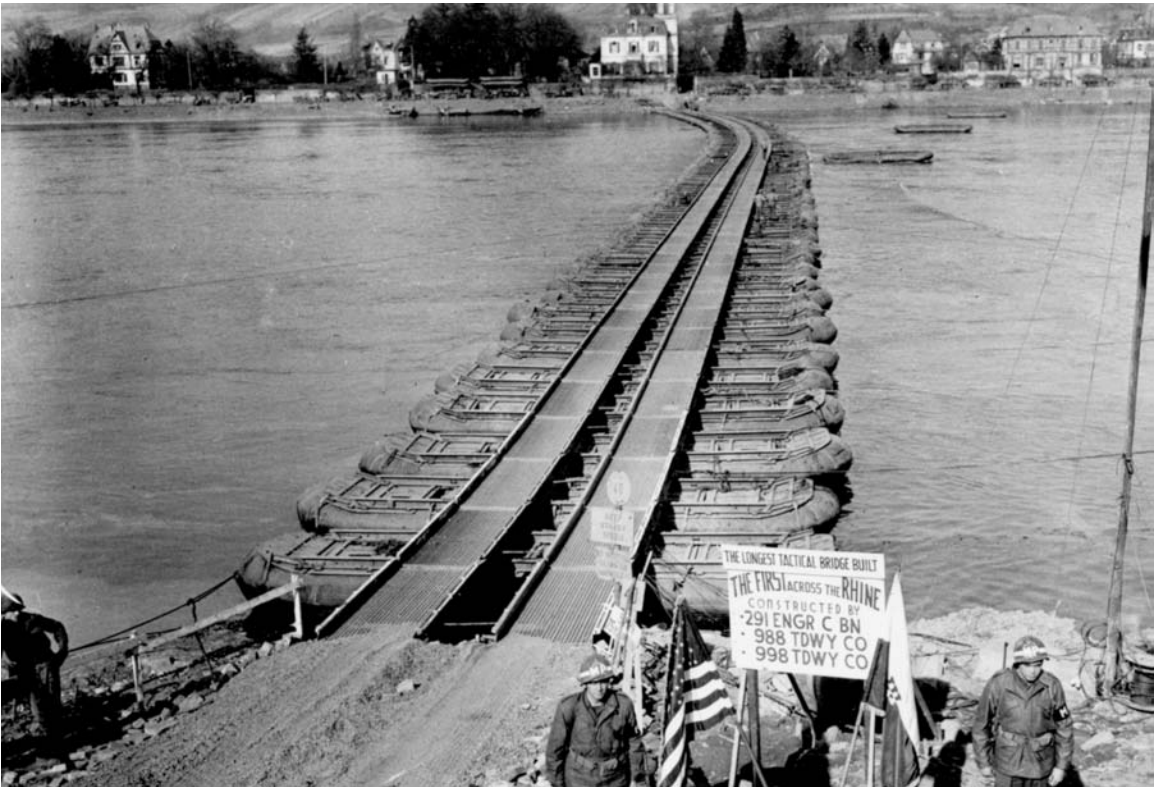
PONTON BOATS AND FLOATS being moved to the Rhine in the Remagen area (top). Treadway bridge across the Rhine near Remagen (bottom). During the period 11–16 March the bridgehead was expanded north and south and all attacks gained ground despite the arrival of enemy reinforcements. Treadway and heavy pontoon bridges were built across the river. As the Rhineland Campaign came to an end, six divisions were east of the Rhine and six more were ready to cross in the First Army zone.
