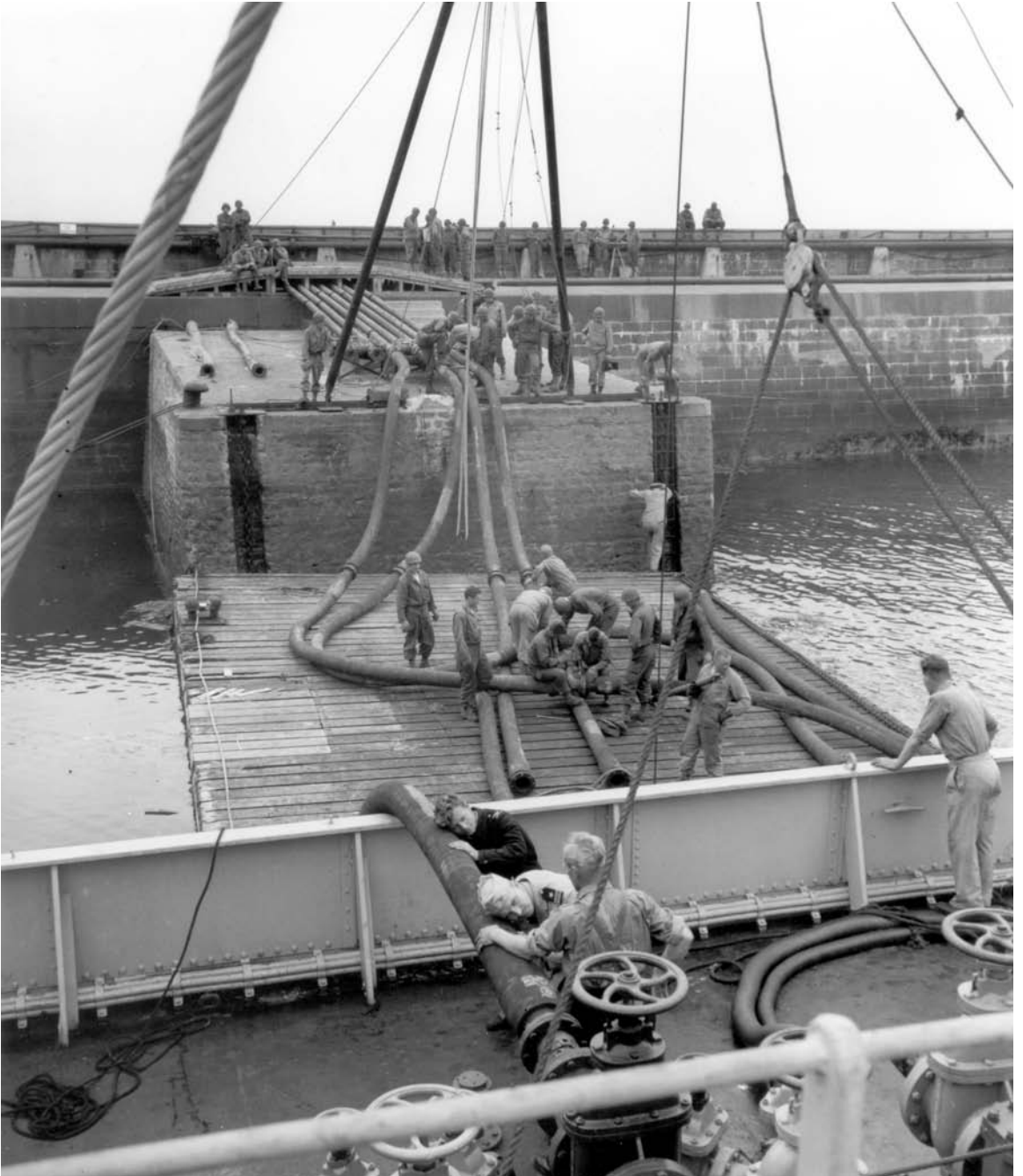
THE FIRST SHIP-TO-SHORE GASOLINE LINE, put in operation at Cherbourg. During the assault phase the Allied forces relied on canned gasoline, but by 3 July bulk supply was being introduced by ship-to-shore pipeline which brought in part of the large quantities of gasoline necessary to the Allied forces.
