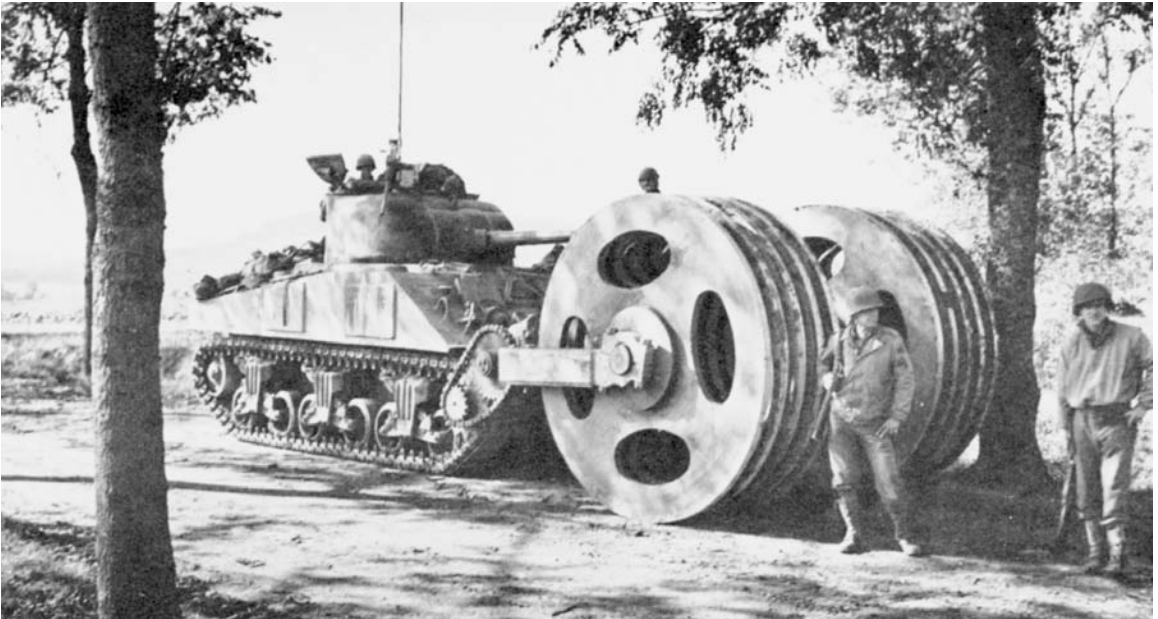
MINE EXPLODER T1E3 attached to a medium tank. This model was an improvement over the earlier one because of its chain-driven exploder disks. On the first models the exploder disks rolled freely and were not power driven. The new model also had a higher degree of indestructibility and greater maneuverability and could be driven in mud eighteen inches deep and across broken terrain. The T1E3 could be driven across a Class 70 military bridge.
