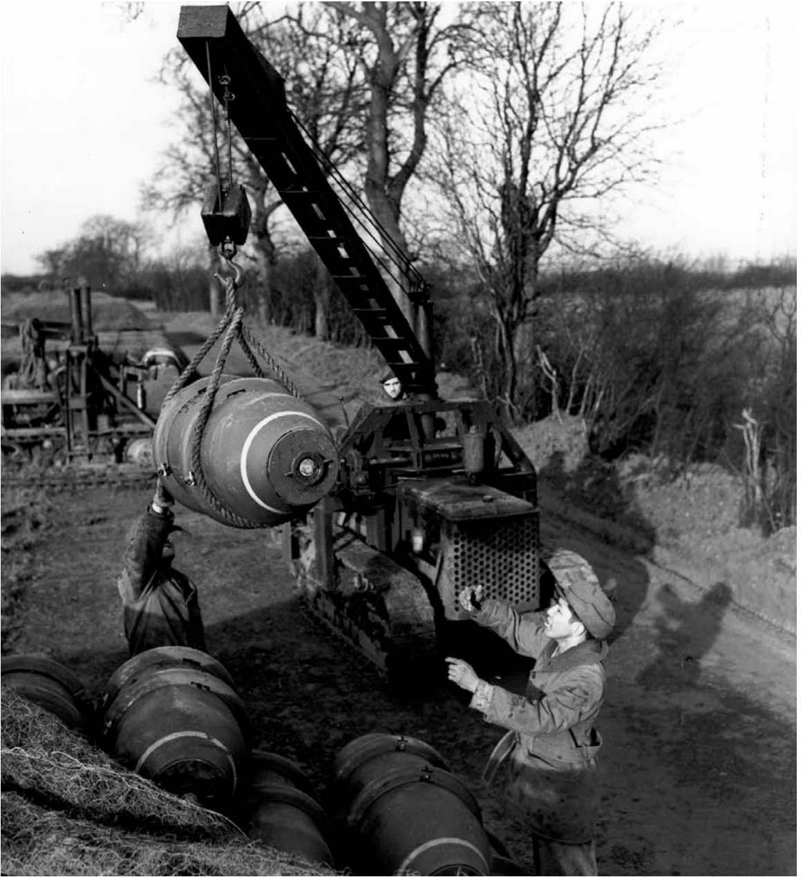
BOMBS BEING UNLOADED at a U. S. Air Corps Ordnance Depot in England. After being stacked the bombs were covered with camouflage nets such as those behind tractors at left center of picture. Facilities for storing bombs in any other manner were limited. These stacks became common sights along the country lanes and roads in England during the war years. (1,000-pound bombs; crawler-type revolving crane on tractor mounting with diesel engine.)
