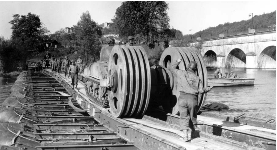
MINE EXPLODER T1E3 attached to a medium tank. This model was an improvement over the earlier one because of its chain-driven exploder disks. On the first models the exploder disks rolled freely and were not power driven. The new model also had a higher degree of indestructibility and greater maneuverability and could be driven in mud eighteen inches deep and across broken terrain. The T1E3 could be driven across a Class 70 military bridge.
