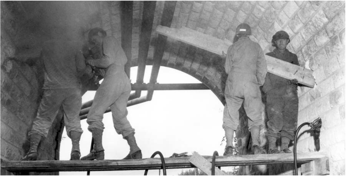
ENGINEERS LAYING A GASOLINE PIPELINE in France. In an effort to transport fuel to the front-line units of the Allies, three fuel pipelines were laid across France. This also relieved the road traffic which became more and more congested as the number of Allied troops in France increased.
