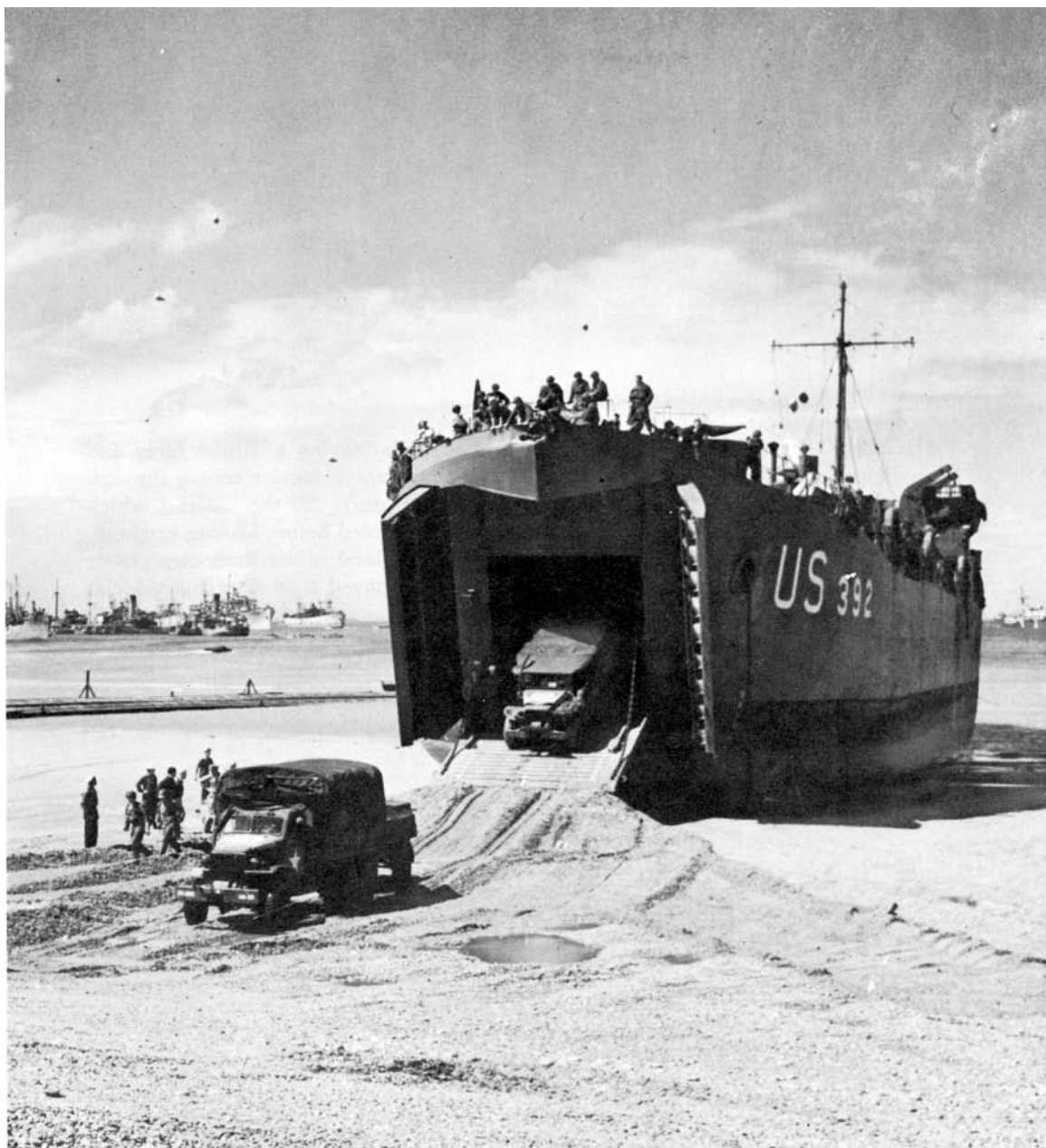
A TRUCK ON THE BEACH (2 \frac{1}{2} -ton) and one starting down the ramp of an LST (1 \frac{1}{2} -ton). After the storm wrecked the artificial harbors emergency measures, such as using 2 \frac{1}{2} -ton amphibian trucks to bring men and supplies ashore and “drying out” landing ships and coasters, were employed. By “drying out” the vessels (as in picture) and unloading directly on the beaches, unloading operations were carried out.
