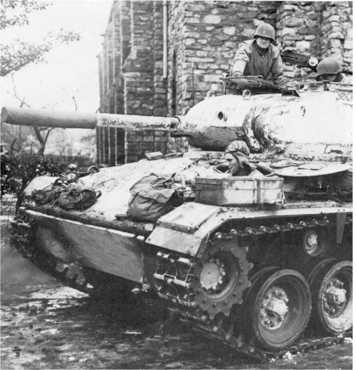
FRONT OF AN M24 LIGHT TANK showing its 75-mm. gun, newer type track, and torsion bar suspension. When the offensive halted attention was given to attacking the Roer dams. The enemy took advantage of the wooded country, deep valleys, many streams, poor roads, and the fortifications of the West Wall in an effort to halt the advance. Bitter fighting developed but by 2 February the U. S. forces had reached a point within two miles of Schleiden. On 8 February the Canadian First Army struck the German forces west of the Rhine, the first of a series of attacks that were to destroy the enemy.
