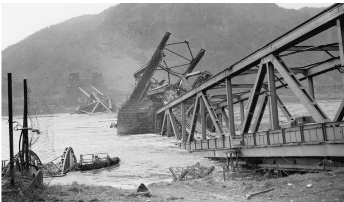
THE LUDENDORF BRIDGE four hours before it collapsed (top). The bridge after it fell into the Rhine (bottom). After capturing the bridge troops were rushed across in pursuit of the retreating Germans while the engineers set to work to repair the damage. Enemy planes made repeated attacks on the bridge and it was shelled by long-range artillery. At 1430 on 17 March the bridge buckled and fell into the river only a few hours before the repairs would have been completed.
