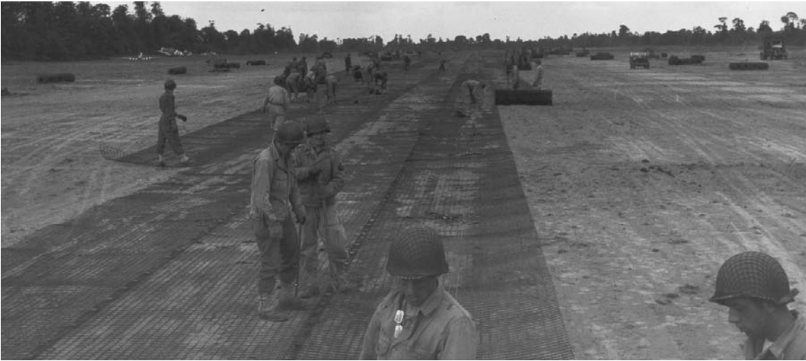
ENGINEERS LAYING WIRE MATTING in the construction of a landing strip near Sainte-Mère-Eglise (top). A Republic P-47 Thunderbolt bursting into flames after crash landing on the strip; still attached to underside of the wing are rockets which were not fired (bottom). An important factor in insuring the success of the Allied close-support operations lay in the establishment of landing strips in Normandy, from which fighter planes could operate. Work began as soon as a footing was obtained on shore and by 9 June planes were operating from these strips.
