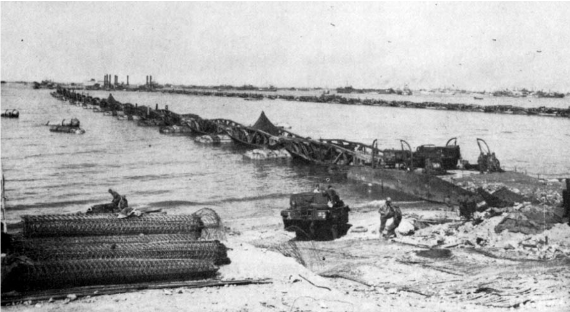
ENGINEERS LAYING STEEL MATTING on omaha Beach at the exits of the causeway which extend to the piers of the artificial harbor (top). Vehicles moving from one of the piers over the causeway to the shore (bottom). These floating causeways to the beach rose and fell with the tide. The artificial harbors were constructed to facilitate the unloading of the large numbers of men and material.
