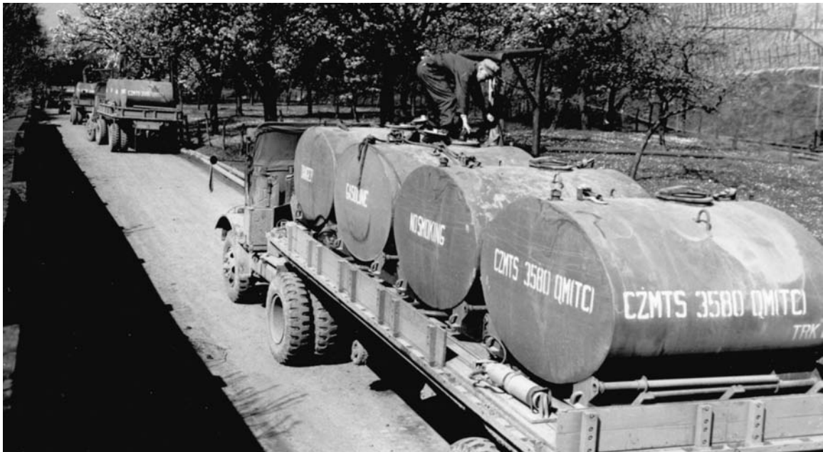
C-47 TRANSPORT, carrying gasoline, lands on an airstrip in Germany (top). Ten-ton semitrailers in Germany with four 750-gallon skid tanks loaded with gasoline (bottom). The versatility of these tanks made it possible to use them on a number of different types of vehicles. During the last months of the war the rapid advances of all the Allied troops made fuel supply a difficult problem. Fuel was transported by every available means to assure the troops an adequate supply.
