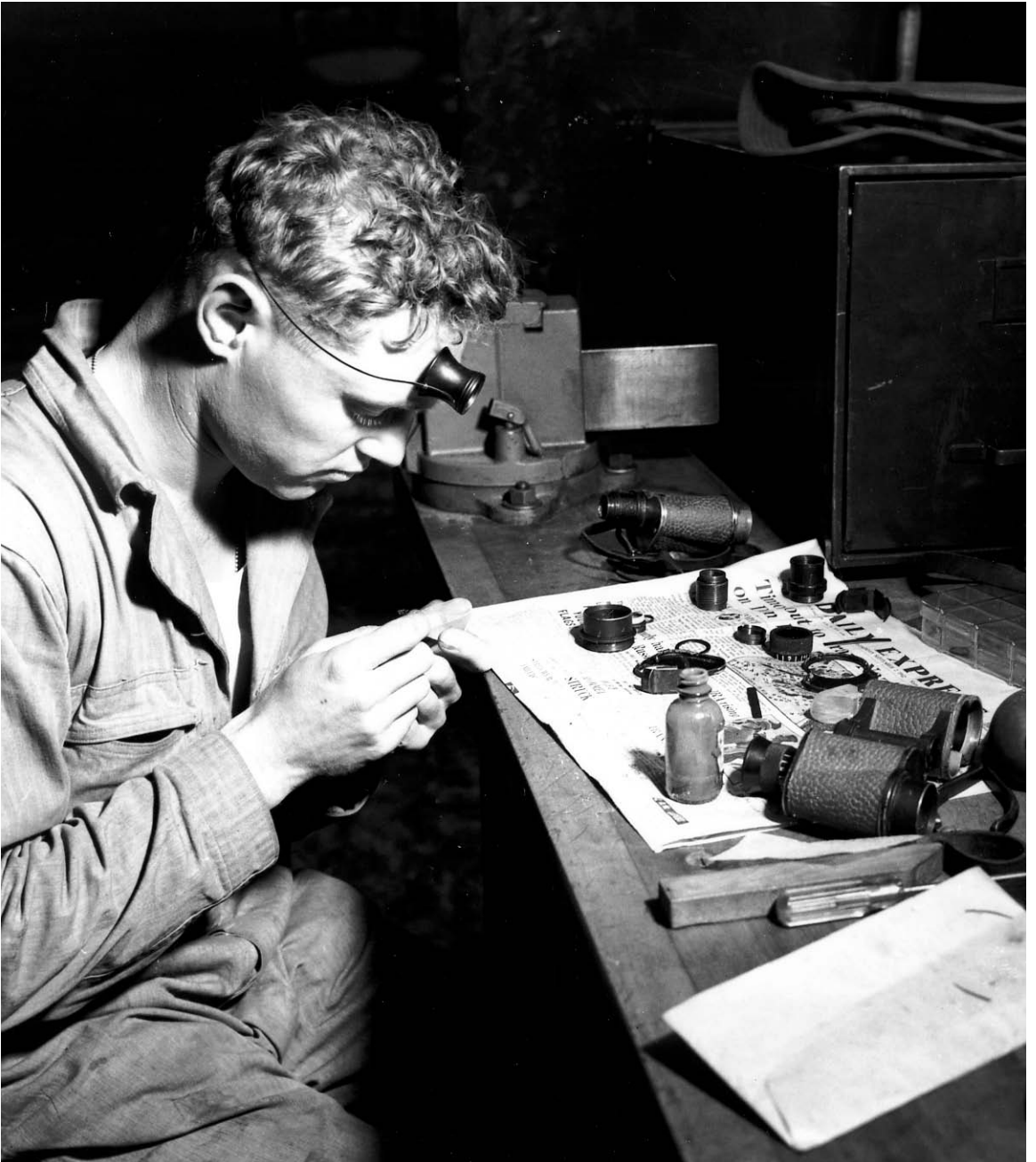
AN ORDNANCE SPECIALIST in the repair of optical equipment cleans a pair of field glasses, England, September 1942. Ordnance responsibility extended to "everything that rolls, shoots, is shot, or is dropped from the air." Its complete catalogue contained 35,000 separate items, ranging from watch springs and firing pins to 20-ton howitzers and 40-ton tanks.
