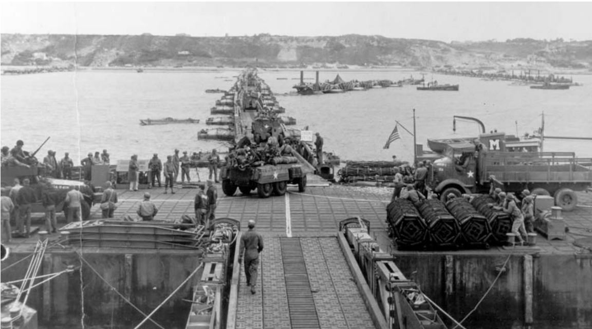
ENGINEERS LAYING STEEL MATTING on omaha Beach at the exits of the causeway which extend to the piers of the artificial harbor (top). Vehicles moving from one of the piers over the causeway to the shore (bottom). These floating causeways to the beach rose and fell with the tide. The artificial harbors were constructed to facilitate the unloading of the large numbers of men and material.
