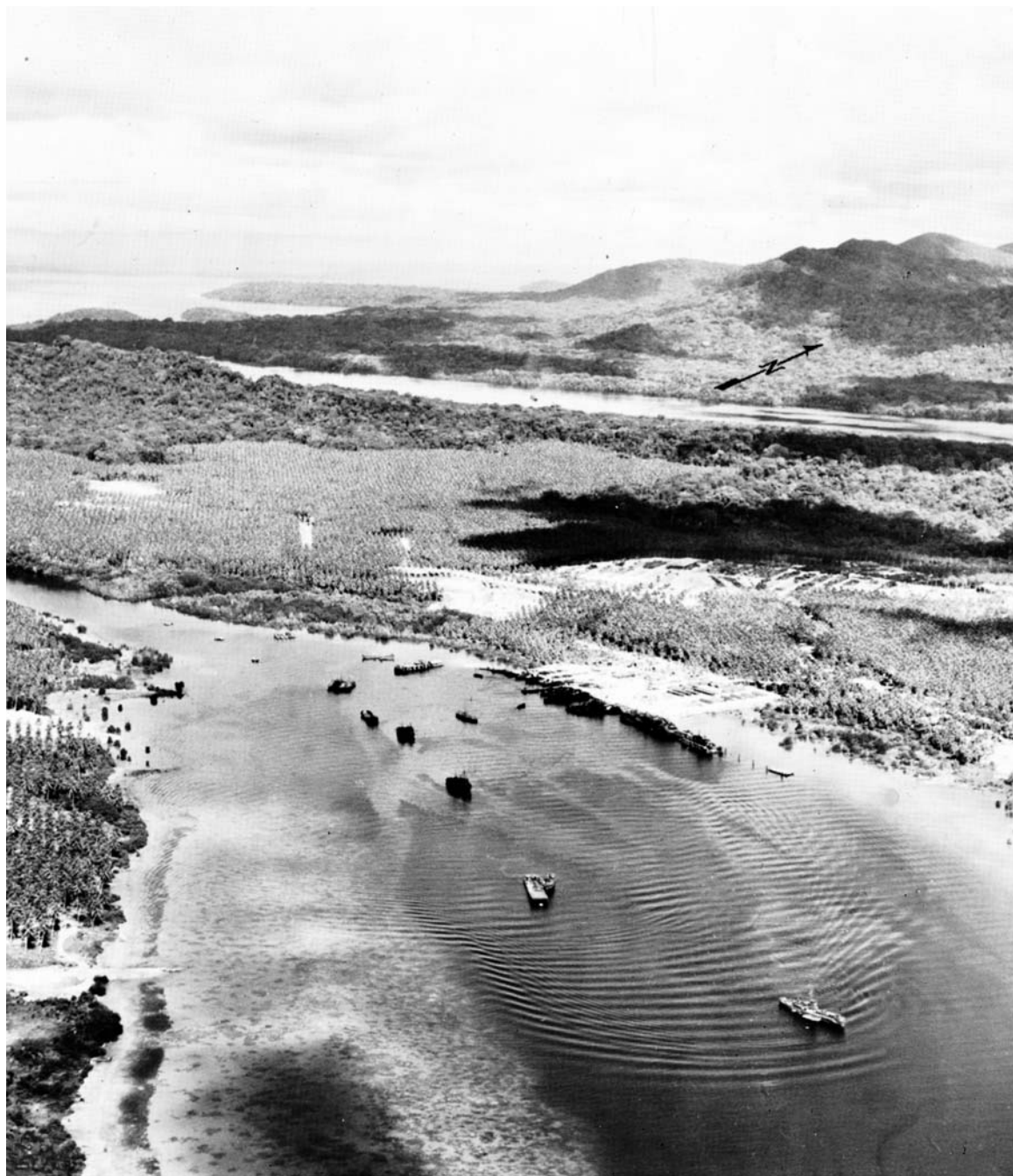
RENARD SOUND, separating the two airfields on Banika. Construction of roads, airfields, and boat bases began in February and by 15 April the first of the two airfields was ready for operation. The torpedo boat base at Lingatu (Wernham) Cove went into operation on 25 February.
