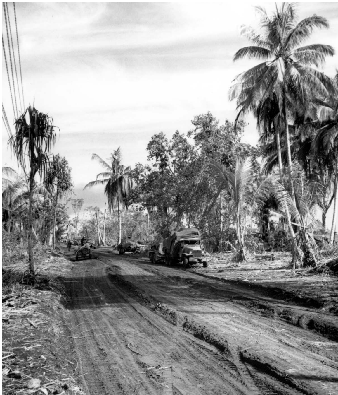
MAIN ROAD AT ARARE being used to transport supplies, 24 May. On 18 May, with artillery support from the mainland, near-by Wakdé Island was assaulted. The next day the large airfield there was taken at a cost of about a hundred U.S. casualties.
