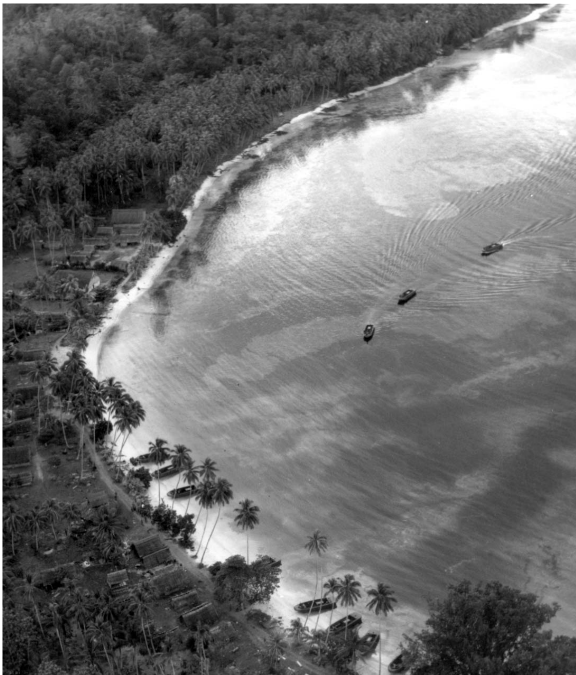
TROOPS LANDING ON FLORIDA ISLAND. Occupation of the island group, Tulagi and its satellites, was accomplished in three days. The enemy garrisons were wiped out except for about 70 survivors who made their way to Florida Island. Mopping-up operations on Florida continued for a few weeks.
