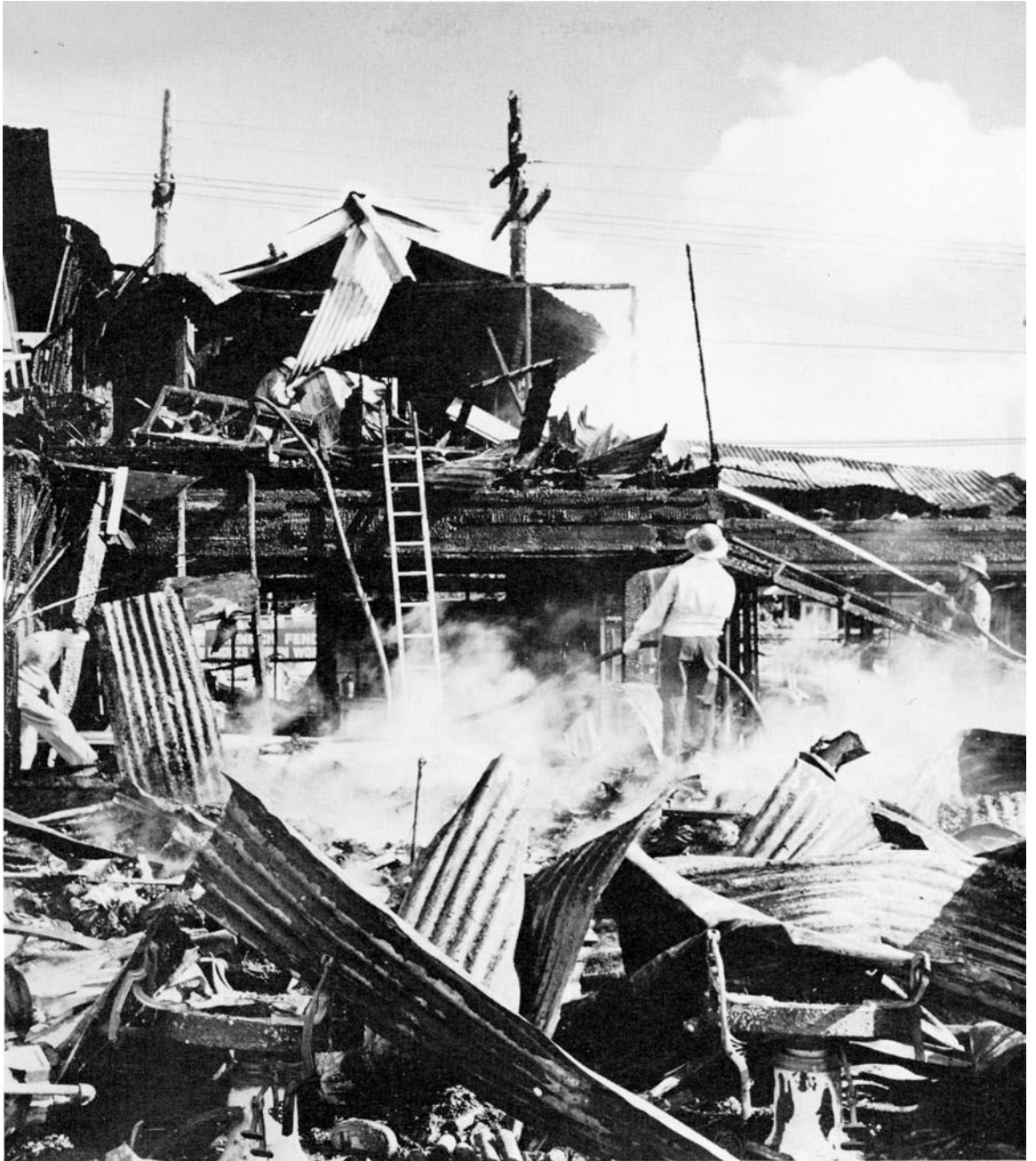
DESTROYED HANGAR AT HICKAM FIELD, 7 December. During the attack the Army lost 226 killed and 396 wounded; the Navy, including the Marine Corps, lost 3,077 killed and 876 wounded. The Japanese attack was entirely successful in accomplishing its mission, and the U.S. forces were completely surprised both strategically and tactically.
