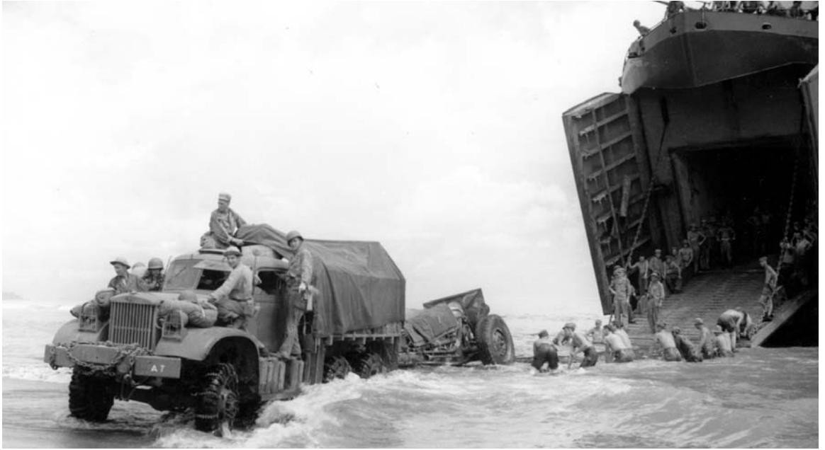
4-TON 6X6 STANDARD TRUCK, with closed cab, towing a 155-mm. howitzer off the ramp of an LST (top); beachhead loaded with ammunition, oil drums, and other equipment (bottom). The barrage balloons over the LST's in the background of bottom picture helped to protect the ships from Japanese dive bombers. Balloons had been let down because of heavy rains. So rapidly were troops and equipment sent in that by the middle of November 34,000 men and 23,000 tons of supplies had been put ashore.
