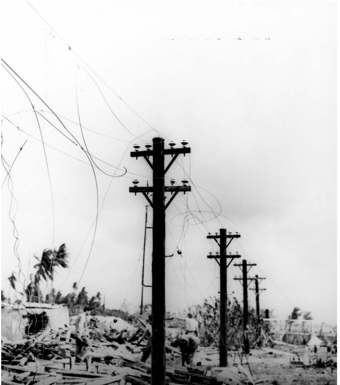
WRECKAGE OF A JAPANESE POWER INSTALLATION found on one of the islands in the Kwajalein Atoll on 31 January 1944. As a result of the air, naval, and artillery bombardment, the islands were greatly damaged. With exception of rubble left by concrete structures, there were no buildings standing; all those which had been made of any material other than concrete were completely demolished.
