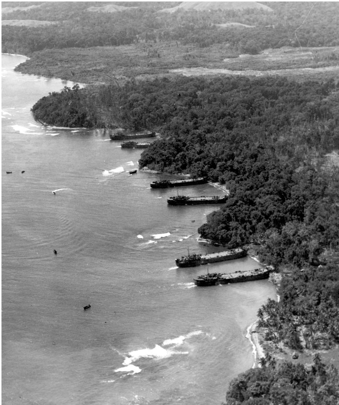
AERIAL VIEW OF SHORE LINE NEAR SAIDOR; ships along the coast are LST's. A regimental combat team landing here had the airstrip at Saidor in use on 7 January.
