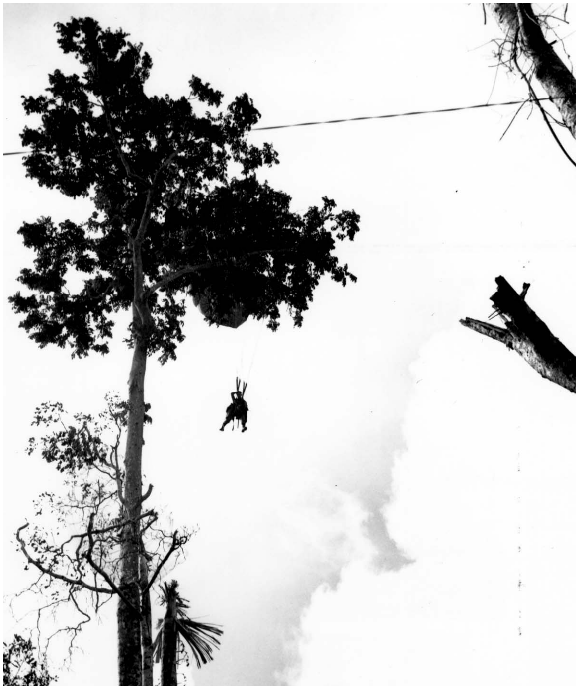
A PARATROOPER HANGING SUSPENDED FROM A TREE in which his parachute was caught during the drop at Noemfoor. All three airfields here were captured by the night of 6 July.
