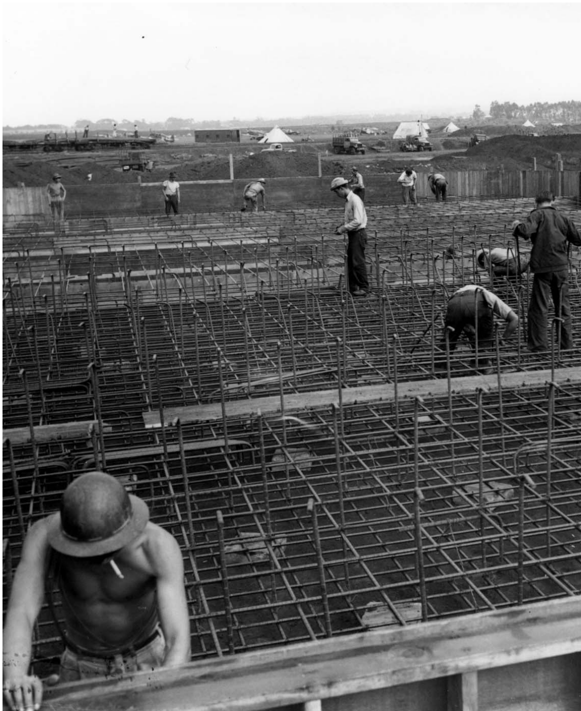
CONSTRUCTION WORK AT WHEELER FIELD, 11 December 1941. After the Japanese raid many destroyed or damaged buildings were rebuilt.
