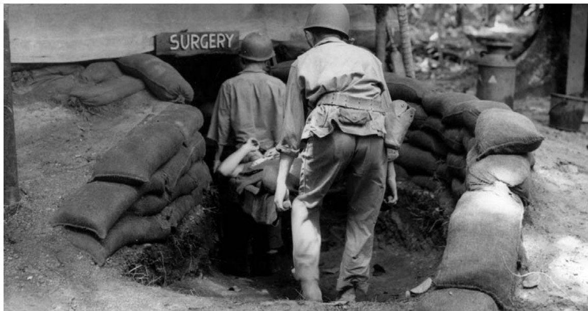
LITTER PATIENT being carried by medical aid men into an underground surgery room (top). Emergency operation being performed in a dugout. This underground surgery room was dug about four feet below the surface and the sides were built up with sand bags and roofed with heavy logs. The entire structure was covered with a pyramidal tent, shielding the occupants from the sun (bottom).
