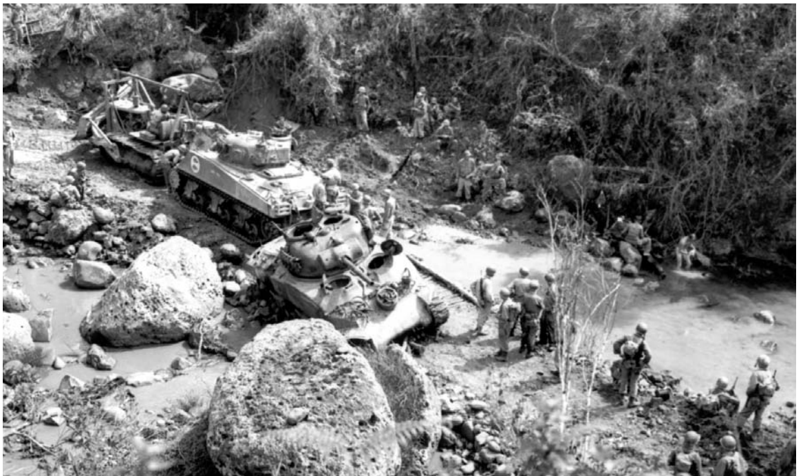
VEHICLES FORDING A RIVER in northern Luzon while engineer troops work on the road; in foreground is a 105-mm. howitzer motor carriage M7. Note destroyed enemy vehicles along road and in stream (top). A bulldozer and a medium tank help another medium tank which has struck a road mine (bottom).
