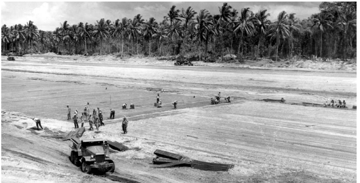
DOUGLAS TRANSPORT C-47 dropping supplies and equipment on an uncompleted airstrip, 30 November 1943 (top); members of a construction battalion laying pierced planking across a runway in the Cape Torokina area, 2 December (bottom). By the end of the year three airfields had been put into operation. The mission of the forces on the island at this time was to maintain a defensive perimeter, approximately ten miles long and five miles deep, guarding installations in the Empress Augusta Bay area.
