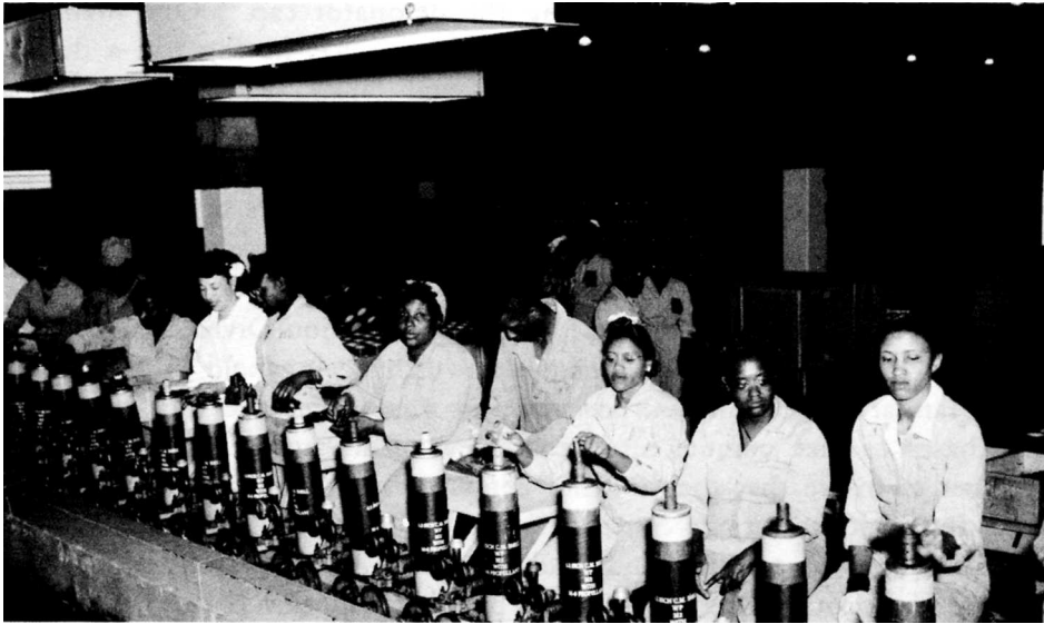
4.2-INCH WP CHEMICAL MORTAR SHELLS on an assembly line, Pine Bluff Arsenal, Arkansas.
