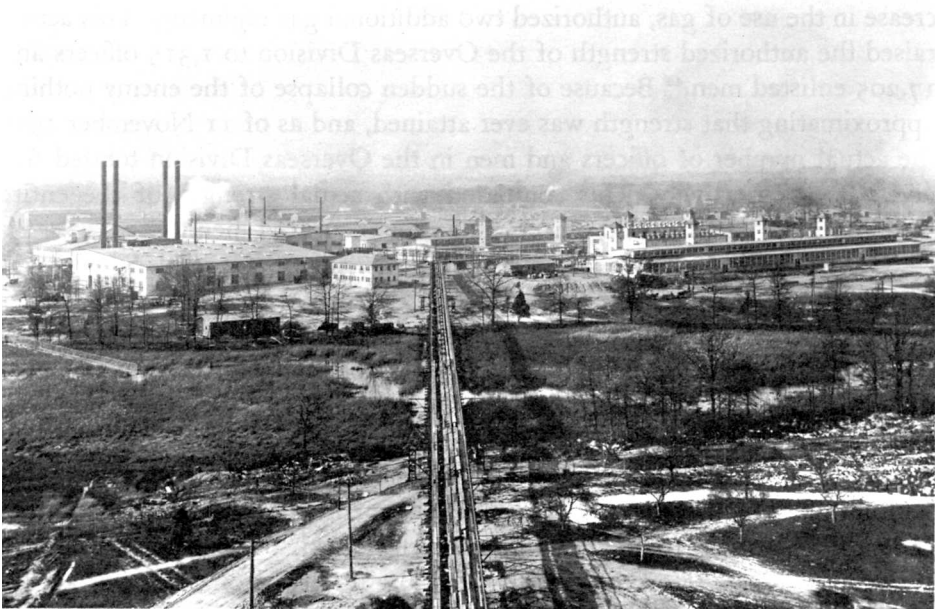
CHEMICAL PLANTS, EDGEWOOD ARSENAL. By 1918, toxic agents totaling 675 tons per week were being manufactured here.
