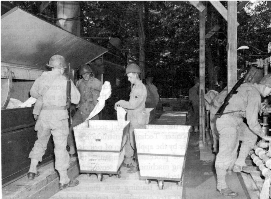
UNIT TRAINING AT CAMP SIBERT. Members of a processing company in field training remove clothing from predryer unit. This is the first stage in the processing of clothing for impregnation. Pipes at lower right carry gas-resistant solution to impregnator unit.
