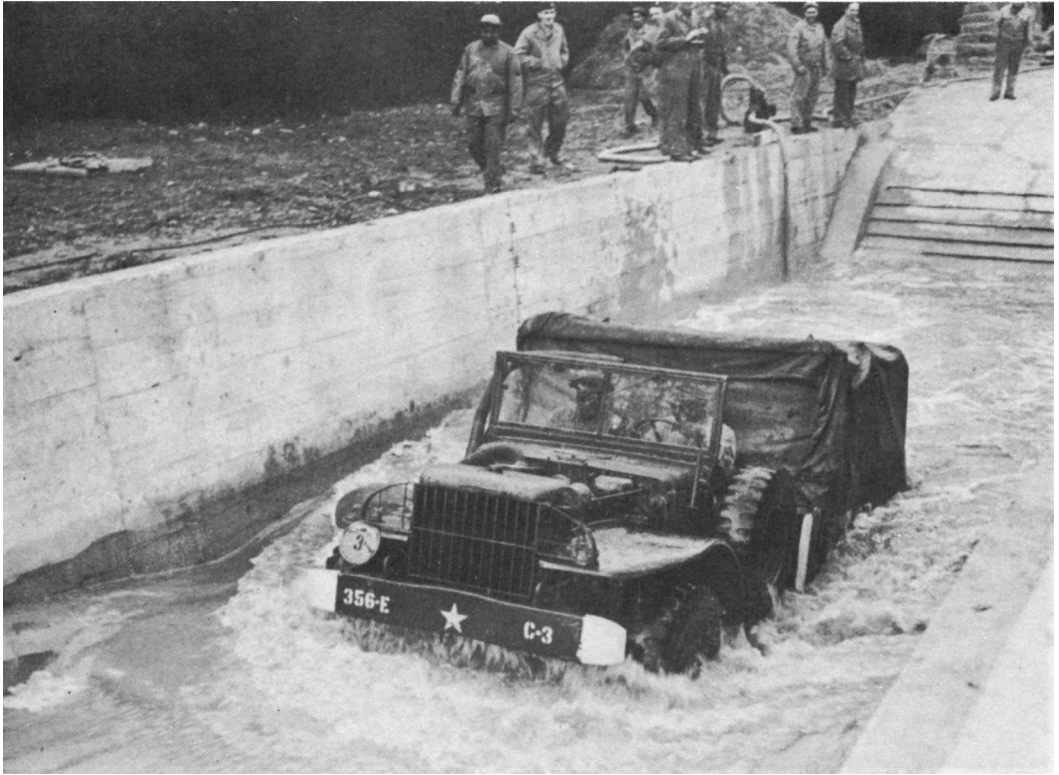
TESTING WATERPROOFED 3/4-TON TRUCK, ENGLAND
