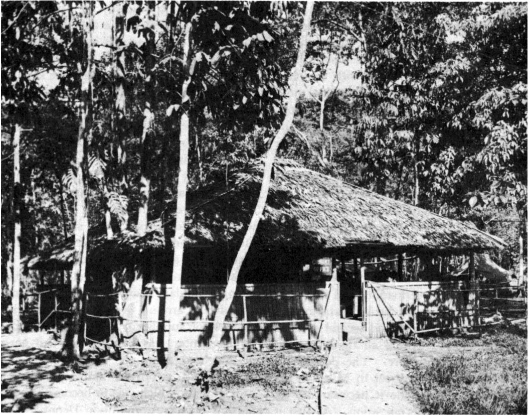
HEADQUARTERS OFFICE, BASE ORDNANCE, ORO BAY, 1943
