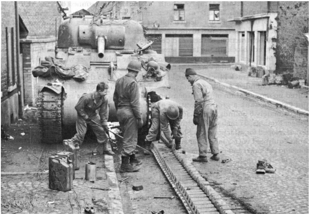
TRACK EXTENSIONS being installed by the crew of a Sherman tank during a lull in combat operations at Baesweiler, Germany.
