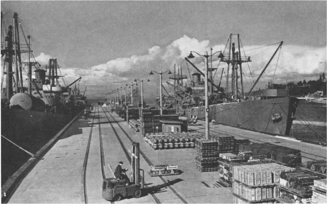
SPECIAL EXPLOSIVES LOADING PIER at Mukilteo, Washington, a facility of the Seattle Port of Embarkation.
