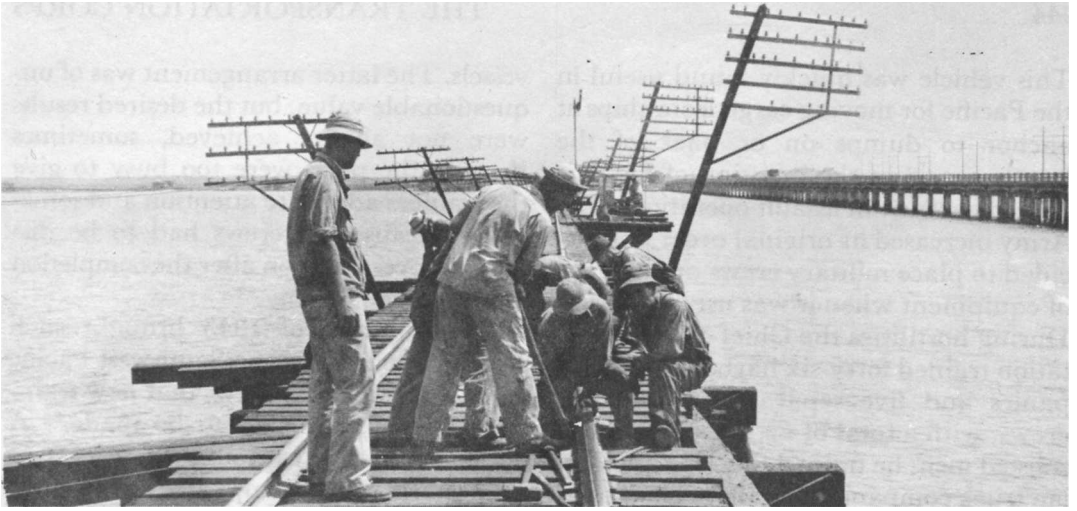
TRAINING TROOPS FOR THE MILITARY RAILWAY SERVICE. Replacements for railway operating battalions repair trestle at Lake Ponchartrain, Louisiana (above). Members of railway shop battalion put on side rod in repair shop at Bucyrus, Ohio (below).
