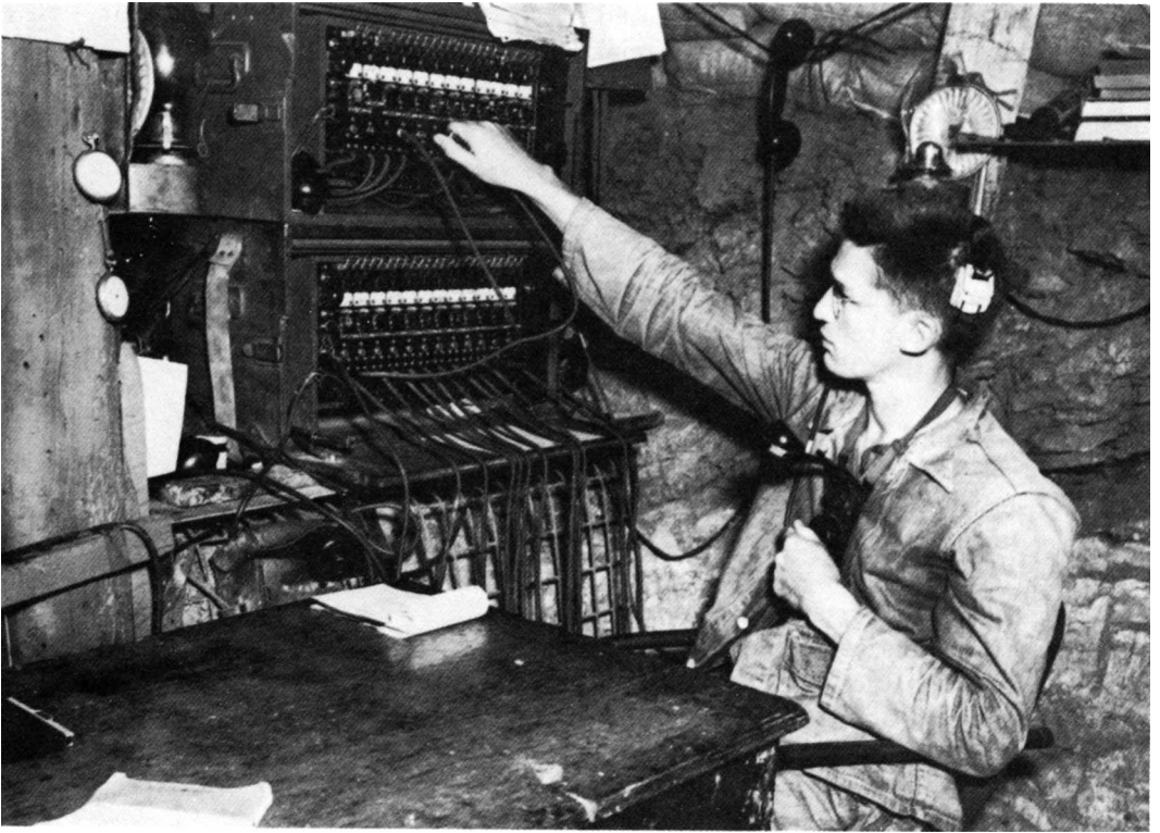
A TWELVE-DROP SWITCHBOARD, the BD-72 , in a communications dugout. ( Photograph taken in 1943. )
