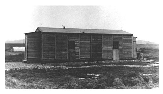
Unit Dispensary at Nome, consisting of two Yakutat huts placed end to end
