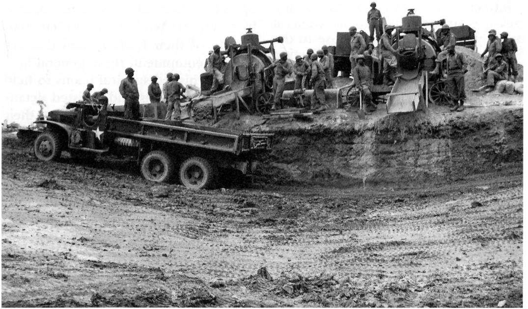
CONSTRUCTING THE 5TH GENERAL HOSPITAL TENTED PLANT AT CARENTAN. Engineers prepare concrete for the ward platforms, and a completed ward tent with beds.
