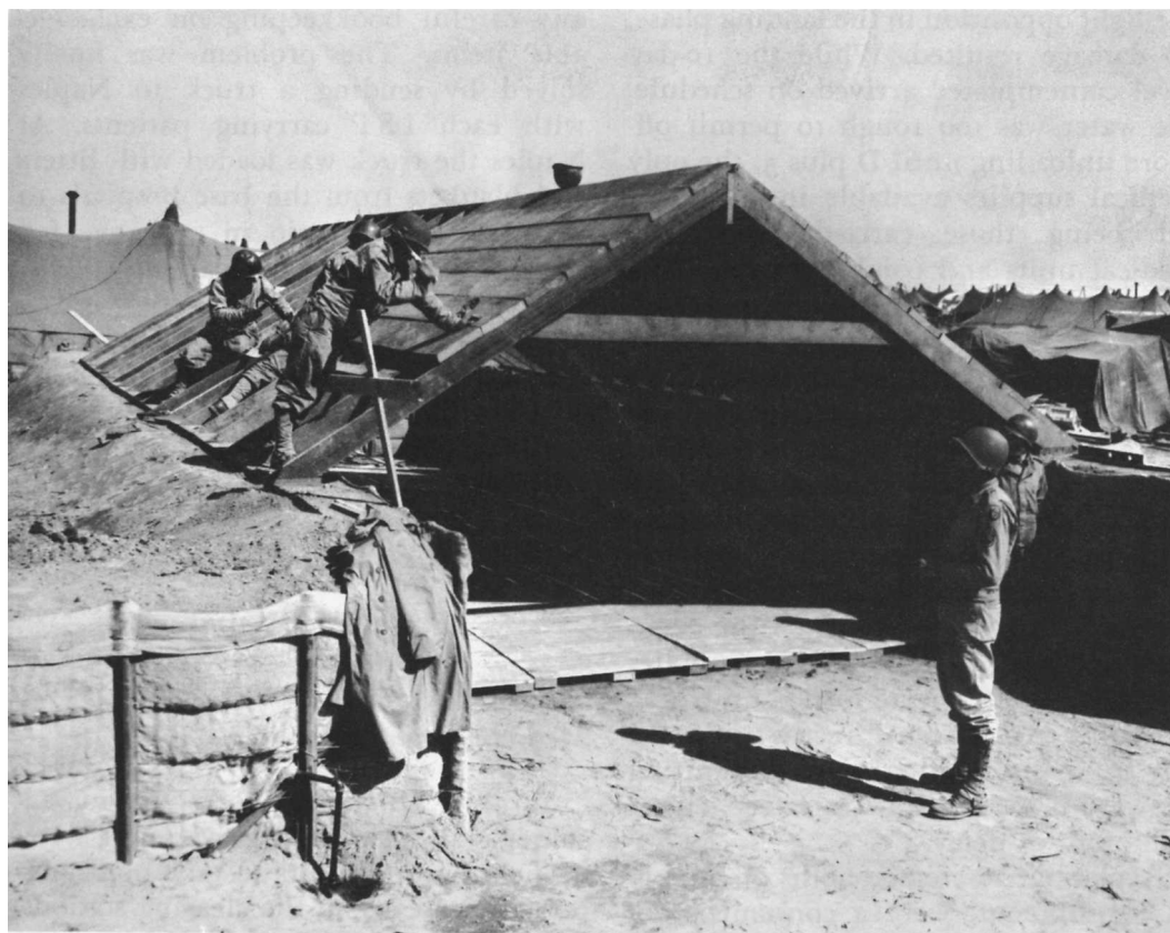
PROTECTING OPERATING TENTS WITH TWO-INCH PLANKS AND SANDBAGS
