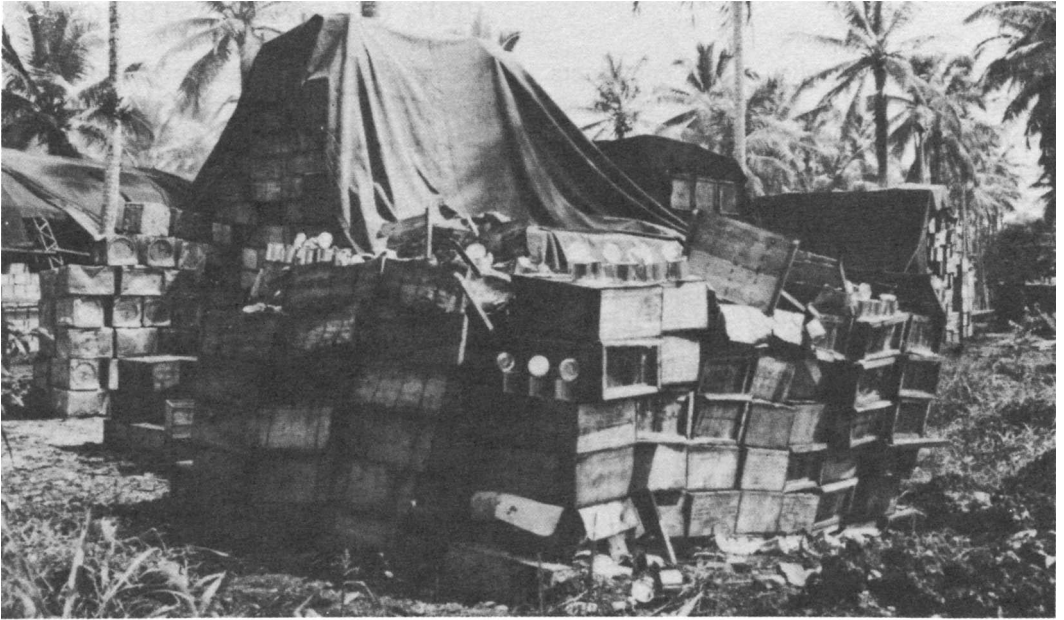
OPEN STORAGE OF QUARTERMASTER ITEMS caused rapid deterioration of outer containers, (above) and lack of dunnage materials forced the use of coconut log ramps (below).
