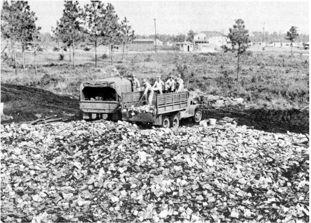
SALVAGE TIN DUMP, Camp Davis, N. C.
