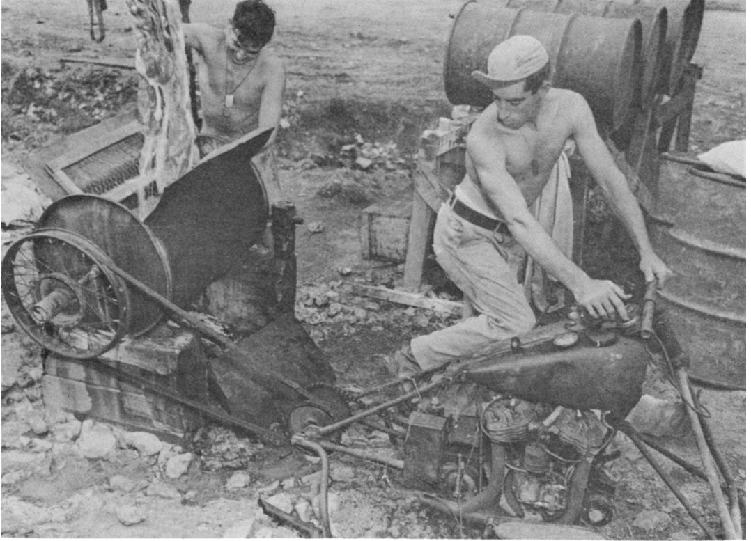
MAKESHIFT WASHING MACHINE built from a steel drum and a motorcycle, Port Moresby, New Guinea.
