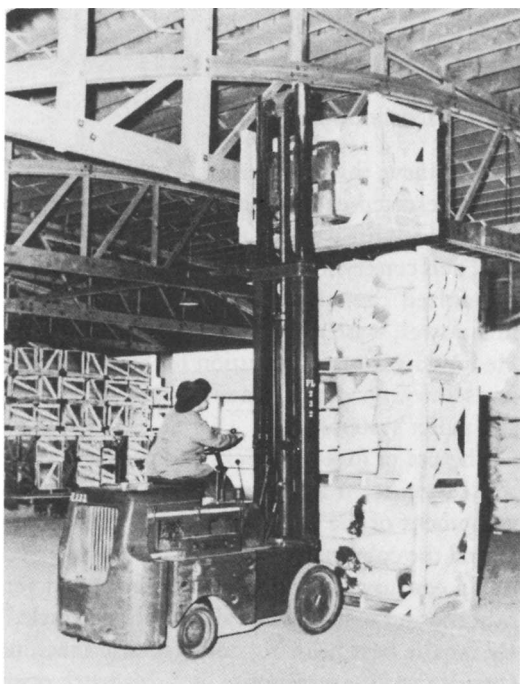
FORK-LIFT TRUCK stacking box pallets (left) and loading a freight car (right).
