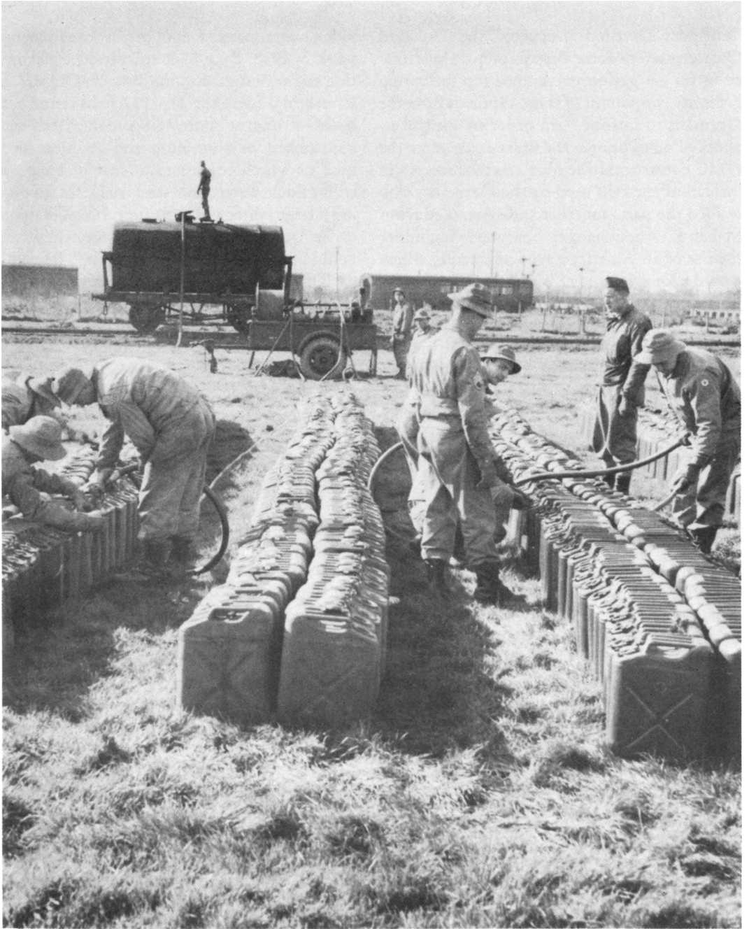
FILLING BLITZ CANS FROM RAILROAD TANK CAR by use of portable gasoline pump.
