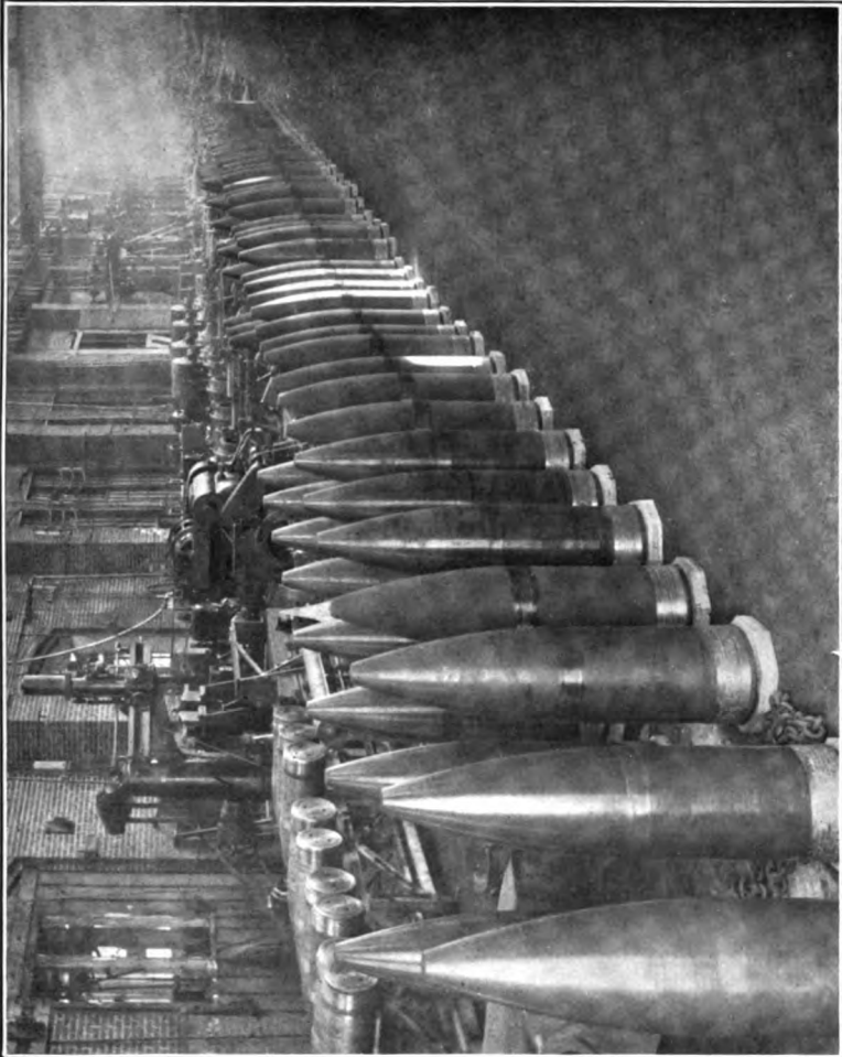
MANUFACTURE OF 14-INCH HIGH EXPLOSIVE PROJECTILES, PREPARED FOR INSPECTION;
