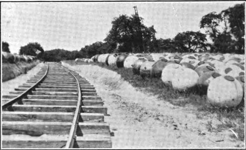
MINES STORED IN THE OPEN AT NAVAL MINE DEPOT, YORKTOWN, VA., AWAITING COMPLETION OF STOREHOUSES.
