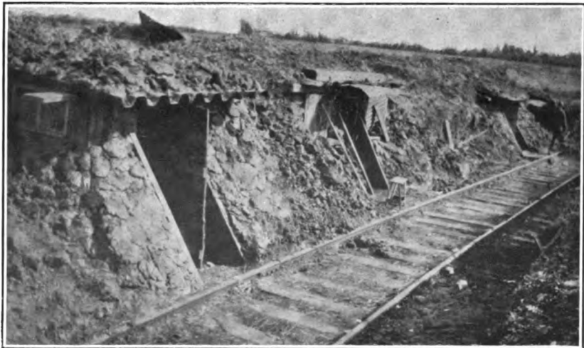
EX-GERMAN BOMB PROOFS OCCUPIED BY NAVAL RAILWAY BATTERY NO. 1, NEAR SOISSONS, OCTOBER, 1918.
