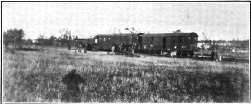
NAVAL RAILWAY BATTERY NO. 1 IN POSITION NEAR SOISSONS, FRANCE.
