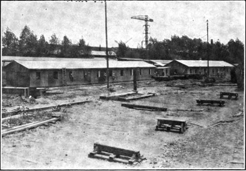
BARRACKS ERECTED BY MEN OF THE U. S. NAVAL RAILWAY BATTERIES. 150-TON CRANE IN THE BACKGROUND.
