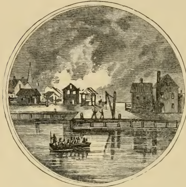
DESTRUCTION AT SODUS BAY.
