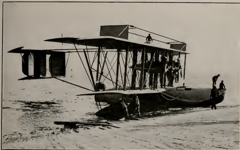
FIG. 21.—SEAPLANE, SHOWING SKID FIN ANTENNA.
