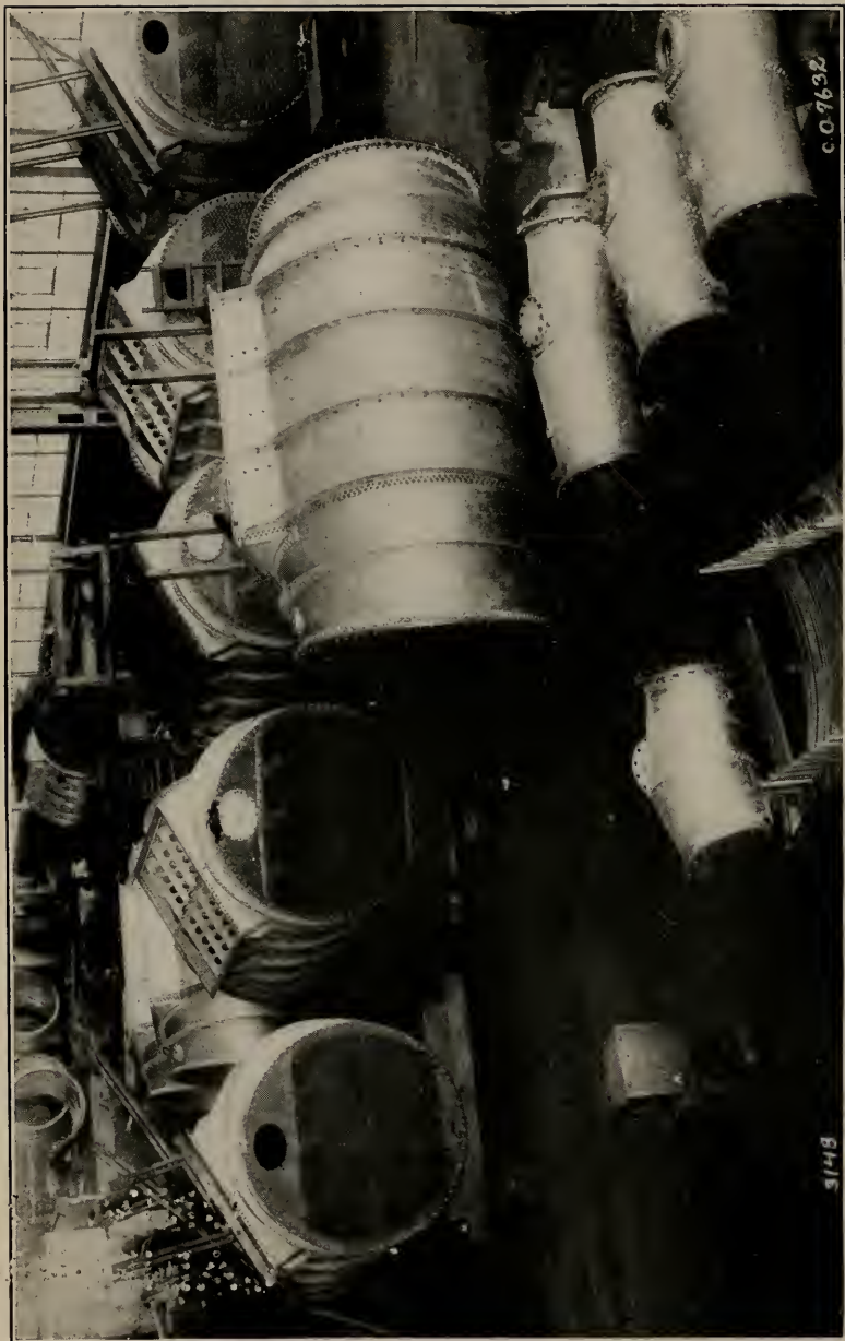
CONDENSERS FOR DESTROYERS. Wellman-Seaver-Morgan Co.
