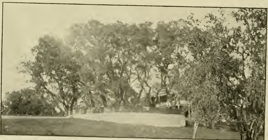
COMMANDER'S RESIDENCE FORT BARRANCAS
