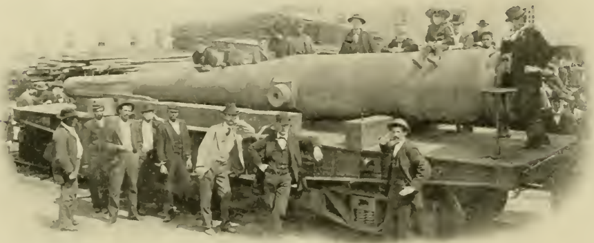
MODERN 50 FOOT GUN BARREL FOR FORT PENSACOLA BEFORE BEING UNLOADED FROM FLAT CAR.
