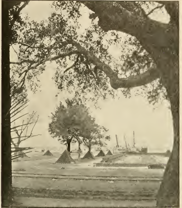
LOOKING SEAWARD, PENSACOLA NAVY YARD
