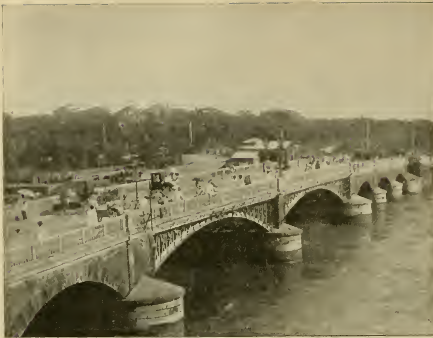
Puerta Espana Bridge Across the Pasig River, Manila
