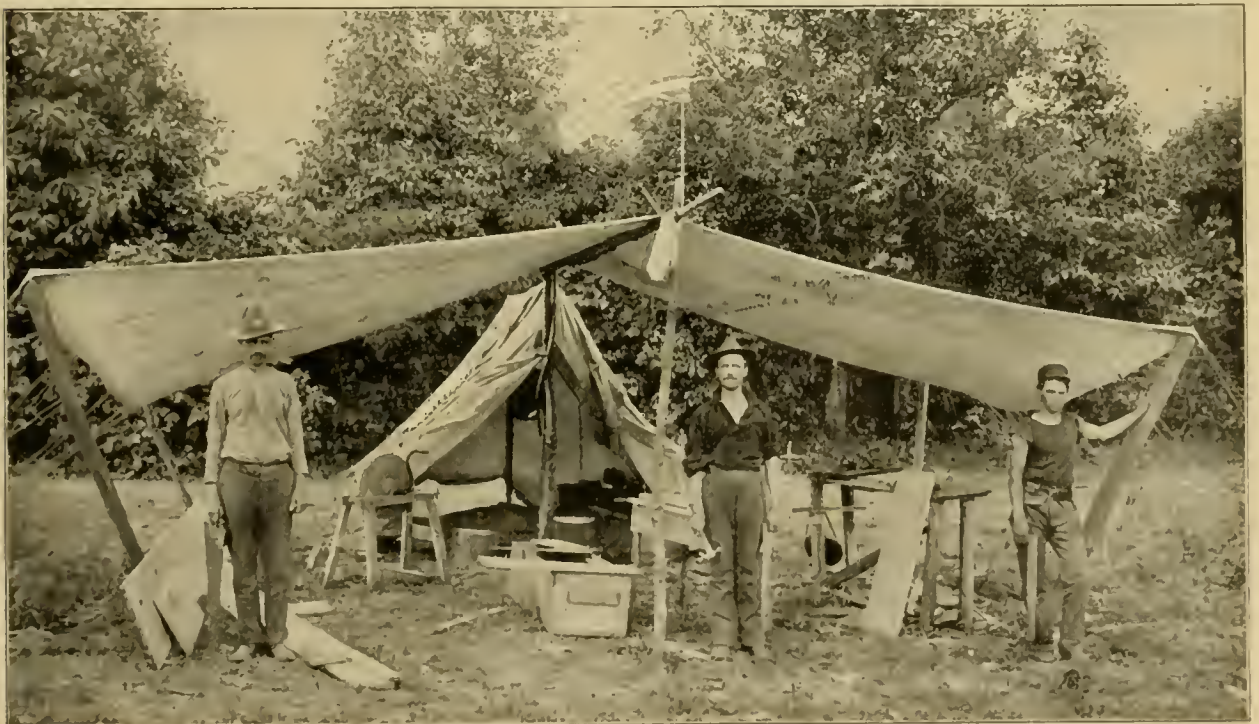
A Regimental Carpenter-shop, at Camp Alger, Virginia
