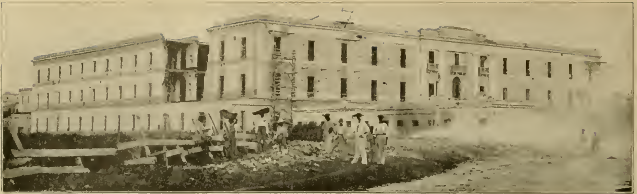
Military Barracks at San Juan—Damaged by American Bombardment
