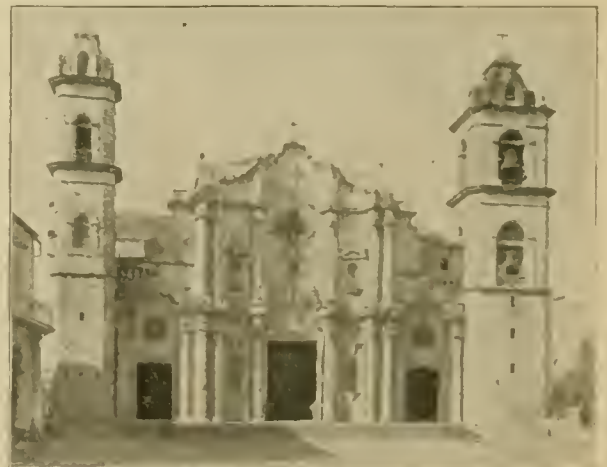
Front View of Cathedral, Havana
