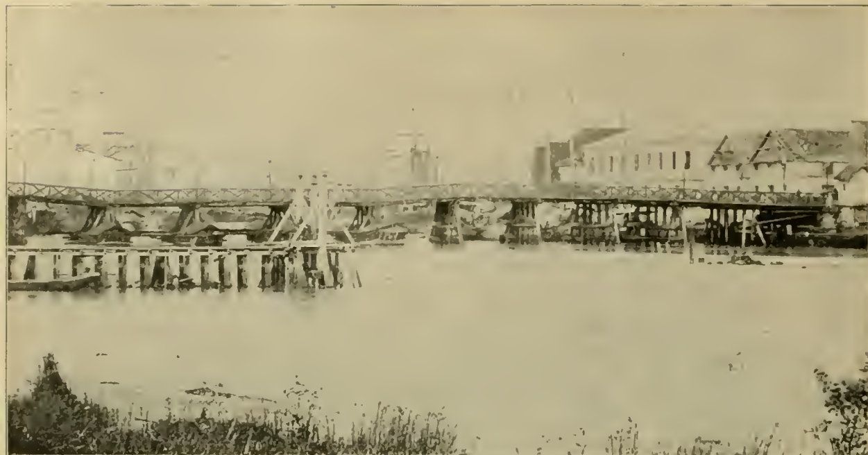
One of the Bridges Across the River Pasig Connecting Old and New Manila
