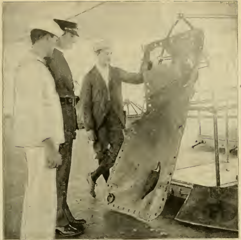
On the Indiana—a Piece of Light Armor Perforated by Spanish Shells
