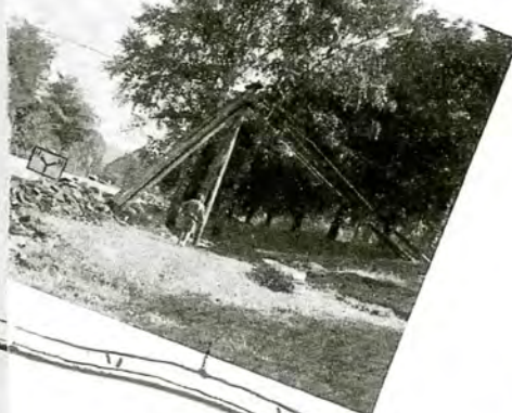
Running cable across the Neckar River
