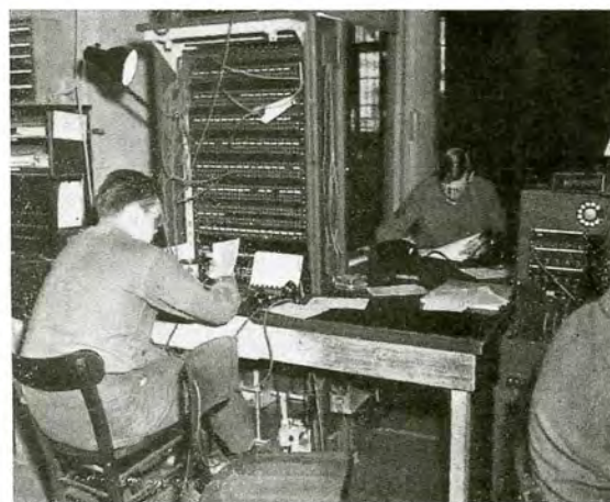
With a tap on every line available, trouble shooting is made a simple operation for wire men
