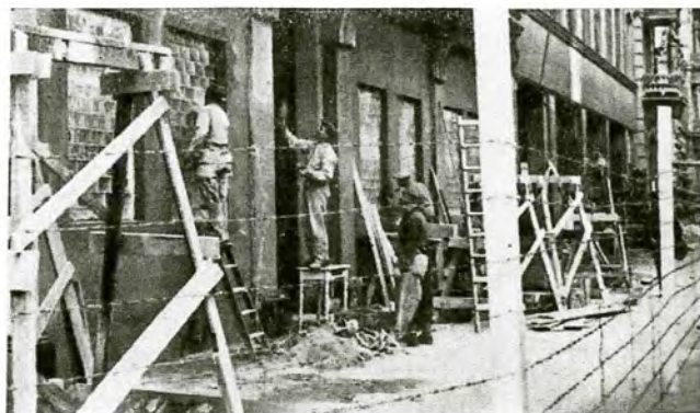
Remodeling of the town in full swing
