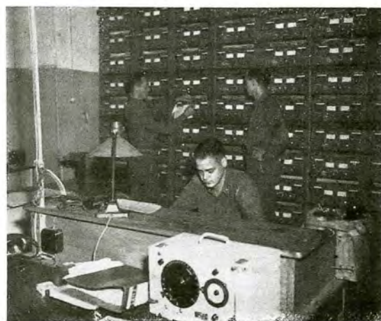
These complicated repeater bays make long distance calls possible to all parts of the American zone
