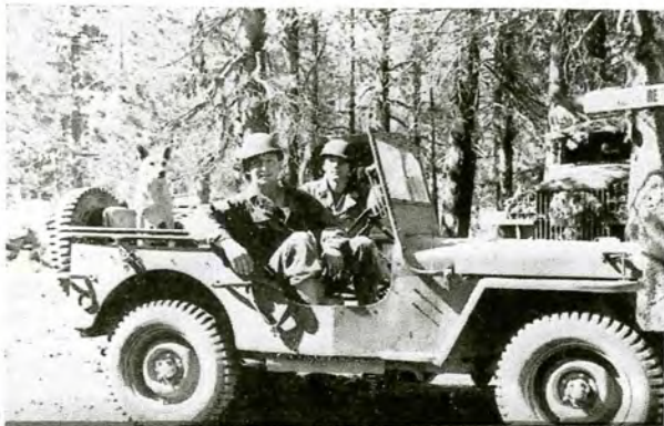
Capt. Costas inspects installation at Lake Tahoe
