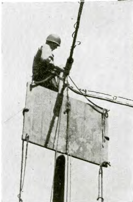
Aerial Cable over the Danub
