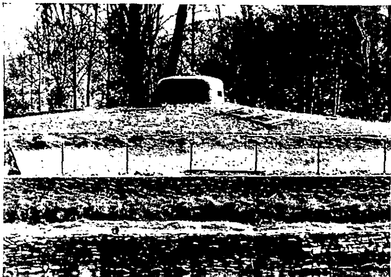
Figure 26.—Work with cupola, embanked.
