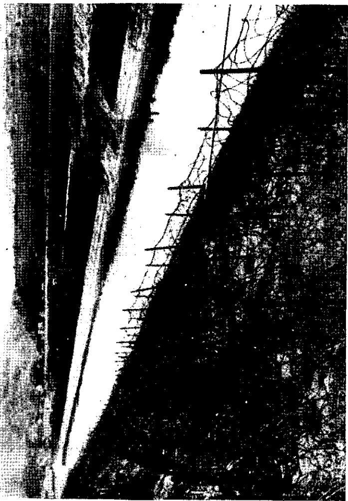
Figure 53.—West Wall anti-tank ditch.
