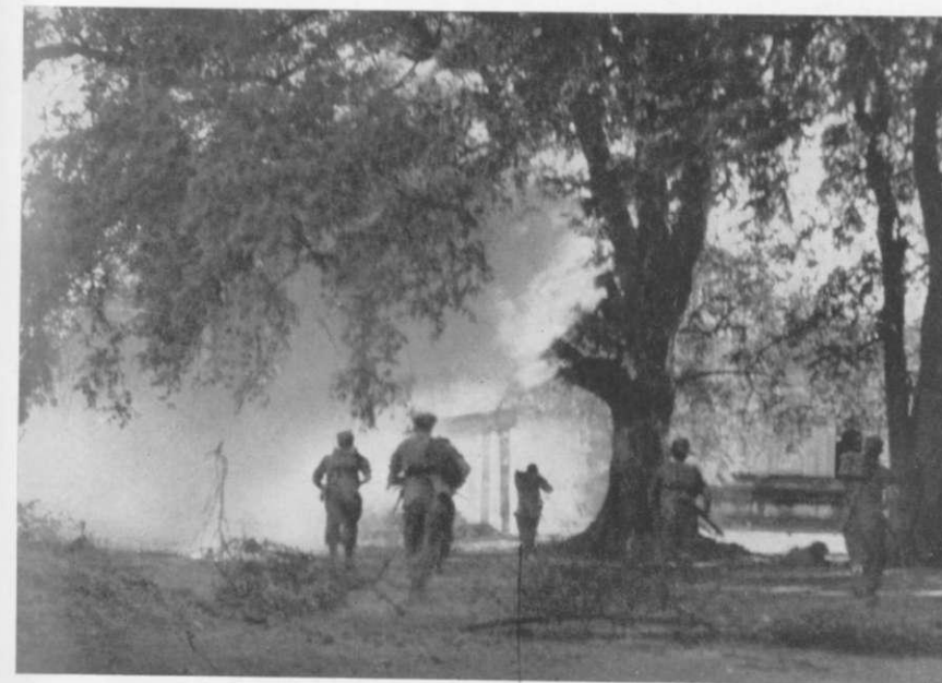
Budalin in flames being attacked
