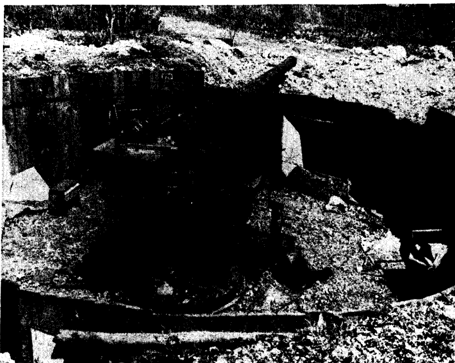
Figure 155.—Type 10 (1921) 120-mm dual-purpose gun (Navy). Note speed-ring sight. The emplacement wall is marked every 45 degrees to speed initial laying.
