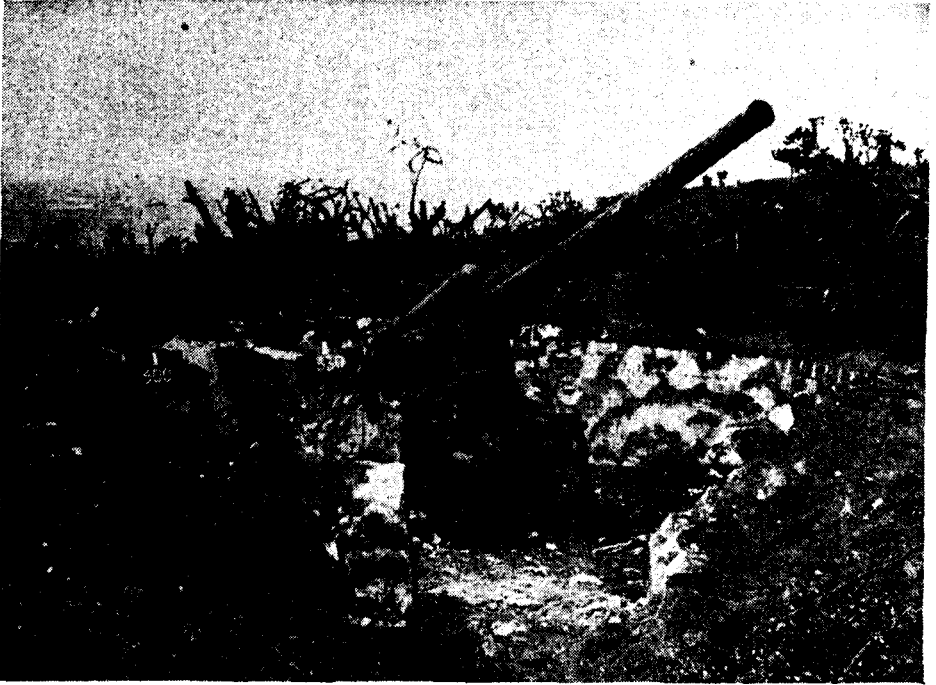
Figure 156.—Type 10 (1921) 120-mm dual-purpose gun (Navy). The emplacement wall is marked for every 5 degrees.
