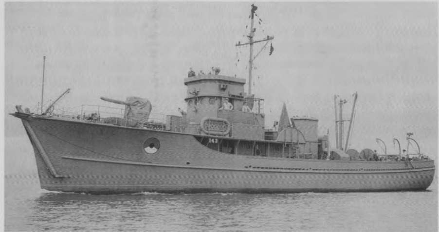
Builder's photograph of motor minesweeper YMS 143, February 1943. As T-522, this ship saw action against Japanese forces on southern Sakhalin Island, 11–25 August 1945. Serving until July 1956, she was stricken from the Soviet navy list and dismantled for spare parts. This type mounted a single 3"/50 cal. gun and two 20mm machine guns, and could make 12 knots.
