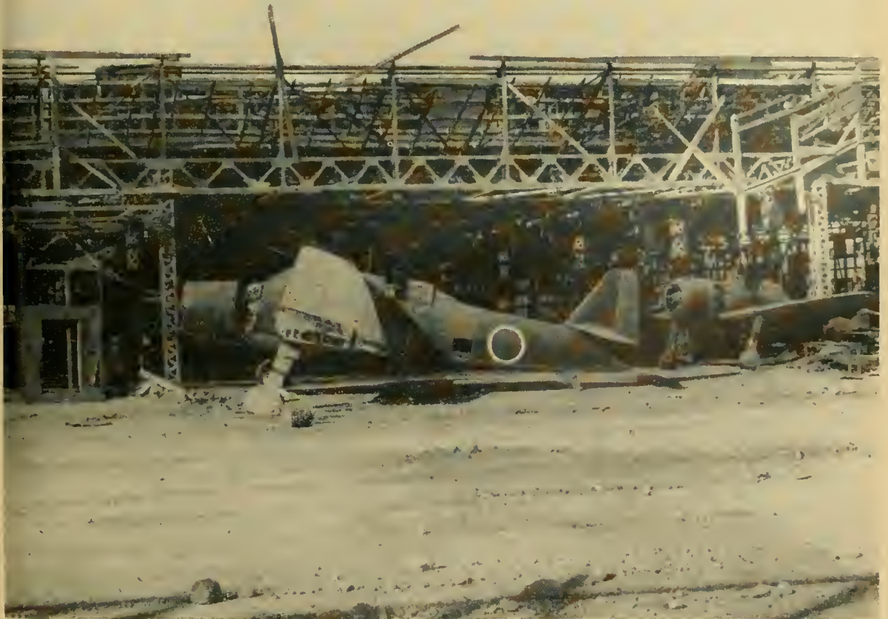
Photo 1: Grace, foreground, and George in front of damaged final aircraft assembly building, Naval Air Depot, Omura
