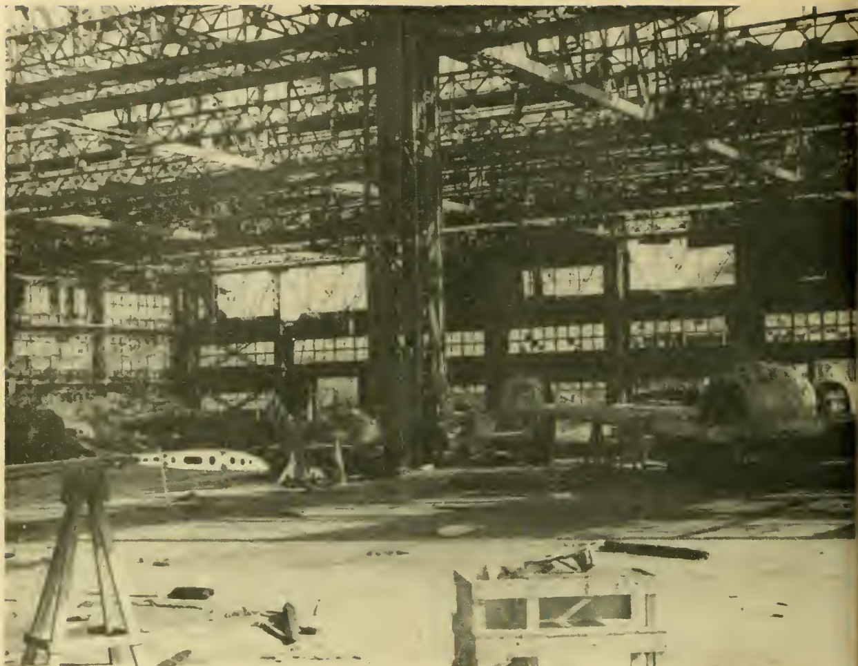
Photo 7: Interior view of damage to No. 1 final assembly shop at Omura
