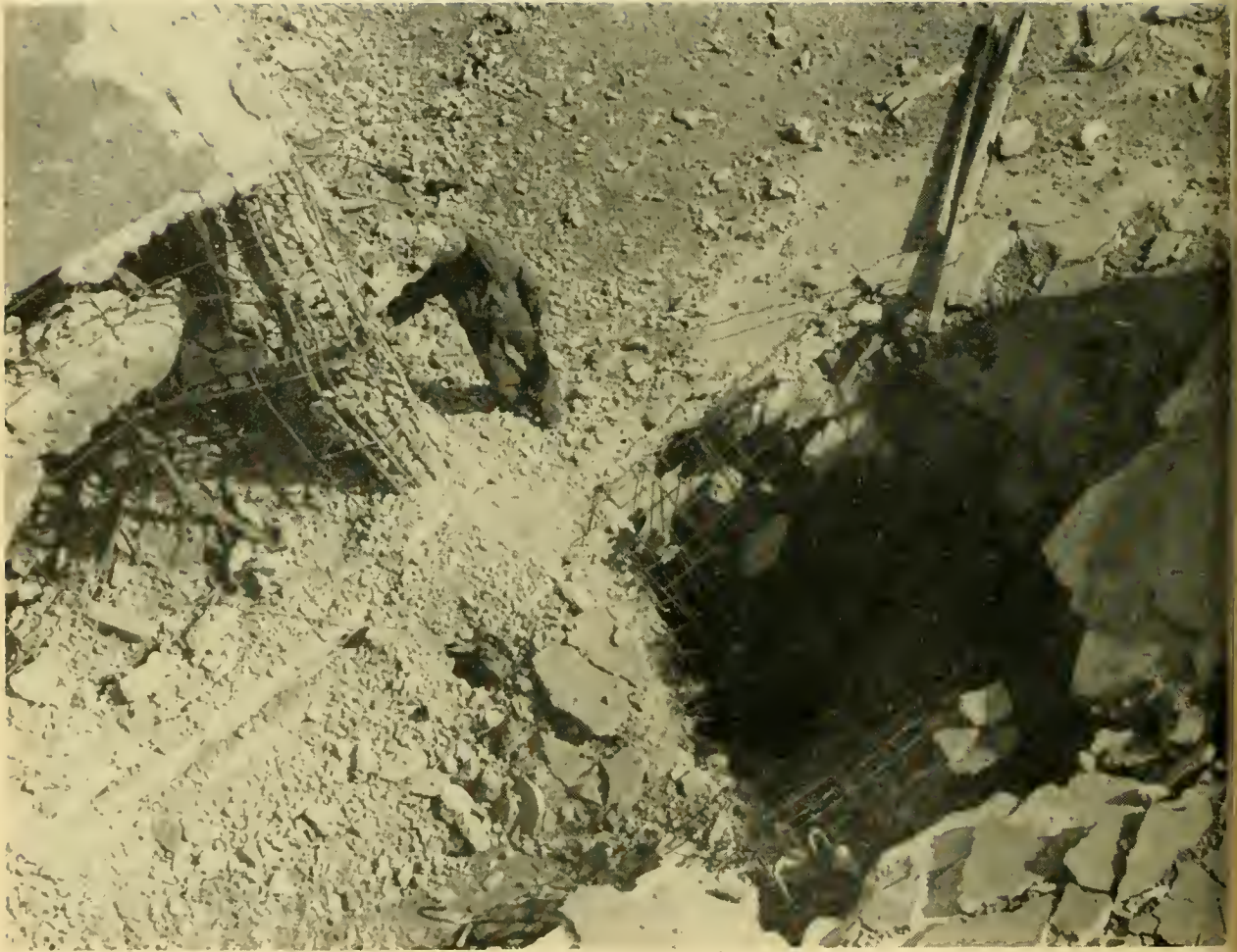
Photo 9: Bomb damage to engine test cells
