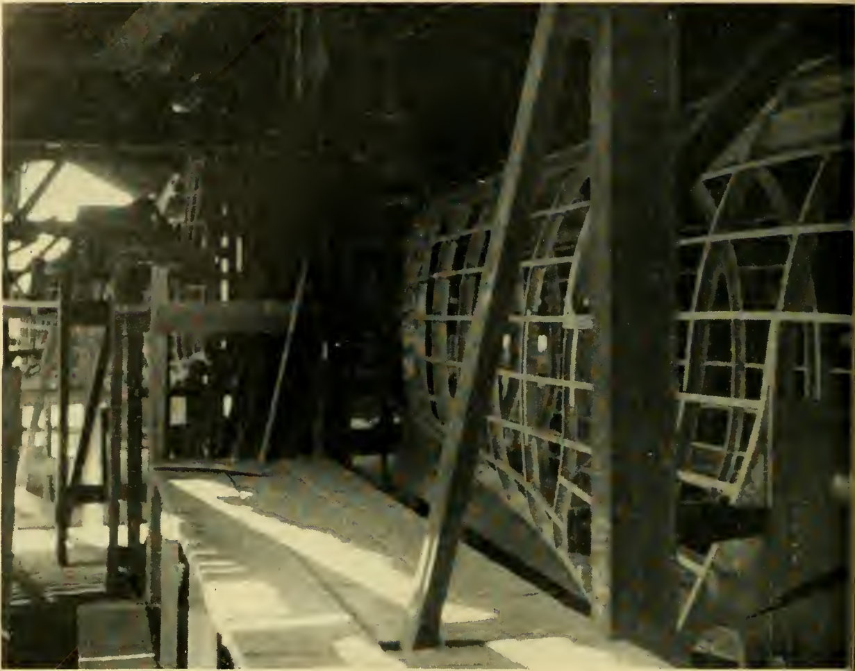
Photo 5: Interior of dispersed George wing assembly shop at Mizubakari
