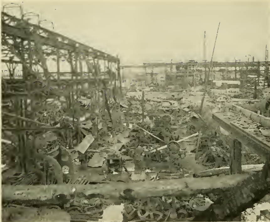
PHOTO 32.—Repair of incendiary damage was frequently regarded as impossible. Lack of electrical cable and fixtures, belting and auxiliary equipment were regarded as greater obstacles than labor and building materials shortages, but damage from exposure was a major factor in reducing the total stock of capital equipment in Osaka.
