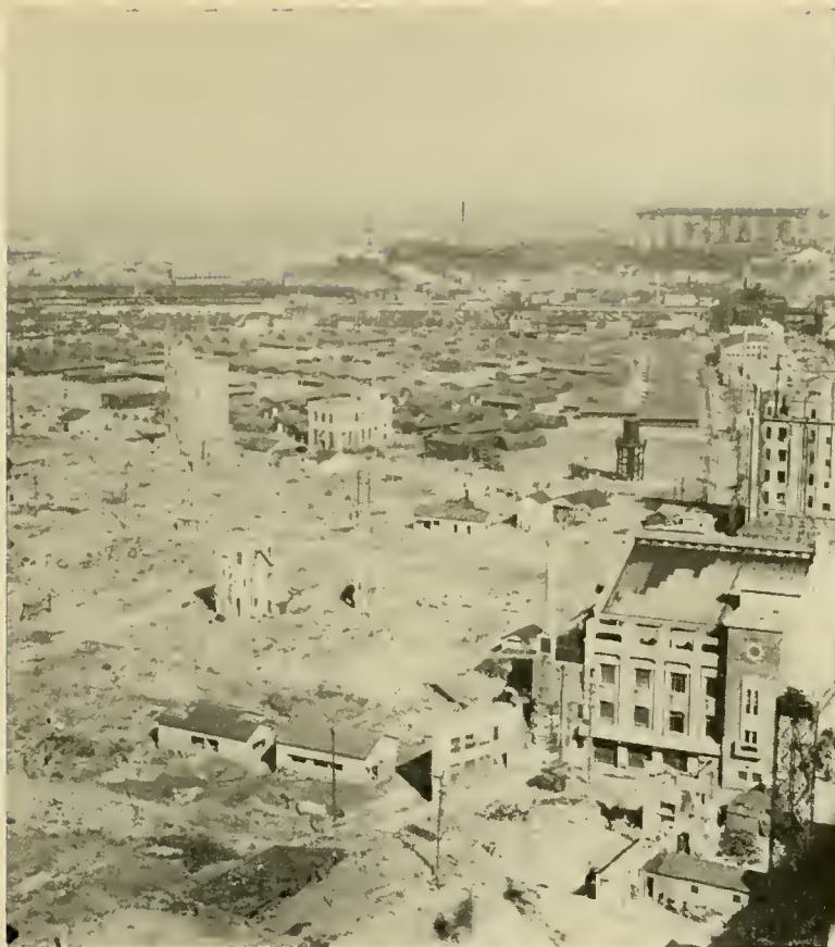
PHOTO 17.—Looking southeast at part of Kawasaki shipyard, where 36 percent of total floor space was destroyed. Quonset huts have replaced satellite workshops, warehouses, and congested workers' quarters in burned-out area around the plant. Even modern concrete structures along thoroughfare leading out of yard suffered considerable damage.
