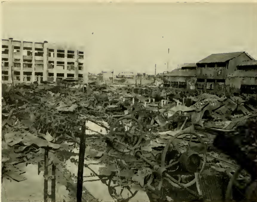
PHOTO 13.—The Nishi district. School building in south industrial district that appeared in aerial photographs to be intact following the March attack. The steel-frame plant on the right was also gutted but appears to be intact.
