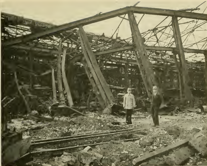
PHOTO 19.—In main assembly section of Kawasaki Rolling Stock Company. An anticlimax to the heavy incendiary damage visible in the background were several high-explosive hits sustained here in July 1945.
