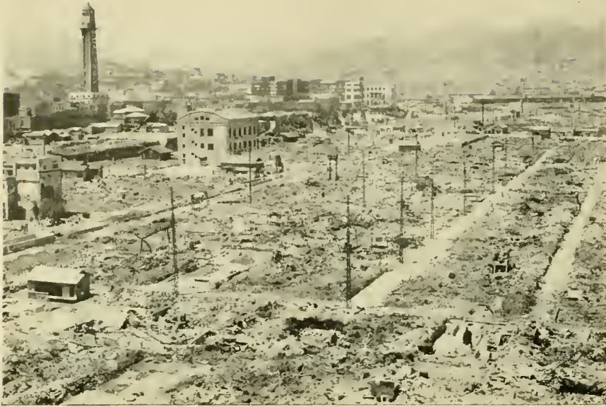
PHOTO 11.—Western Kobe. Looking northwest toward upland outskirts near edge of area destroyed in June incendiary attack. Group of small machine shops in foreground was completely burned out and scrap equipment was only partially removed. Modern fire tower was one of few concrete structures in photo where building contents were not destroyed.
