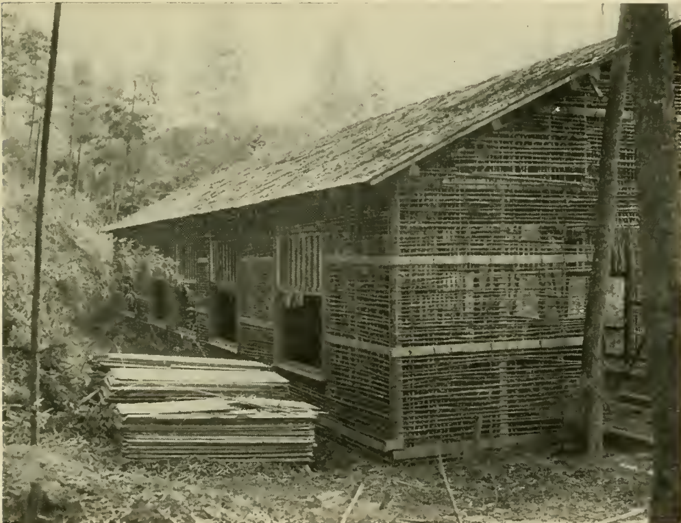
PHOTO 29.—Close-up of unfinished dispersal structure showing typical Japanese construction methods for small factories and shop buildings.
