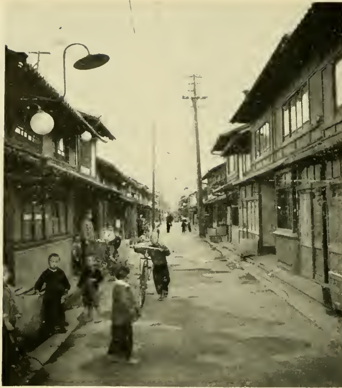
PHOTO 2.—Typical street in Kyoto. Except for a few main thoroughfares, street widths are like this in commercial as well as residential districts. Operatives of small workshops and stores pictured here customarily live on upper floors. Structures are of wood and stucco construction and are directly joined. This pattern is typical of that which prevailed in large sections of most Japanese cities.
