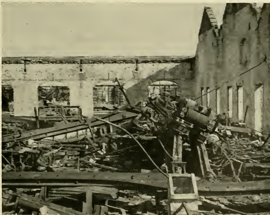
PHOTO 15.—Other sections of the Takatori car repair shops. Collapse of roof girders and traveling cranes prevented salvage of any equipment.
