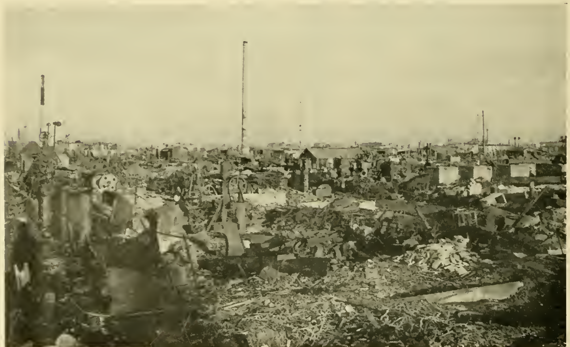
PHOTO 12.—The Minato district. A closer view of gutted machine shops in the same district pictured in Photo 11. Construction was uniformly wood, composition, and sheet metal throughout this section. Damage dates from the 1 June attack. Note shacks built by former residents out of salvaged sheet metal.
