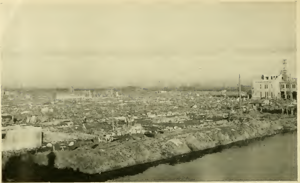
PHOTO 11.—The Minato district. Looking northeast toward Osaka castle across almost eight miles of uninterrupted destruction. Photo taken from center of densely populated southwest industrial district. Concrete firehouse was gutted but remained standing.
