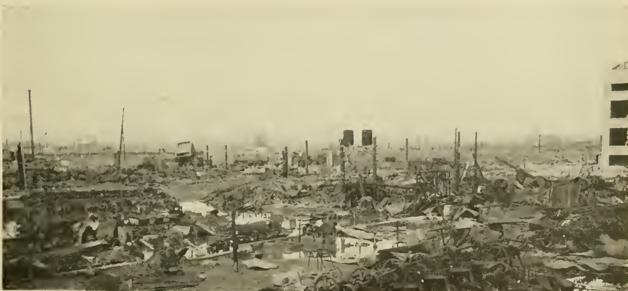
PHOTO 25.—Post-attack view in same district. Except for occasional concrete structures, only burned-out transformers and industrial debris mark the location of former small factories and workshops.
