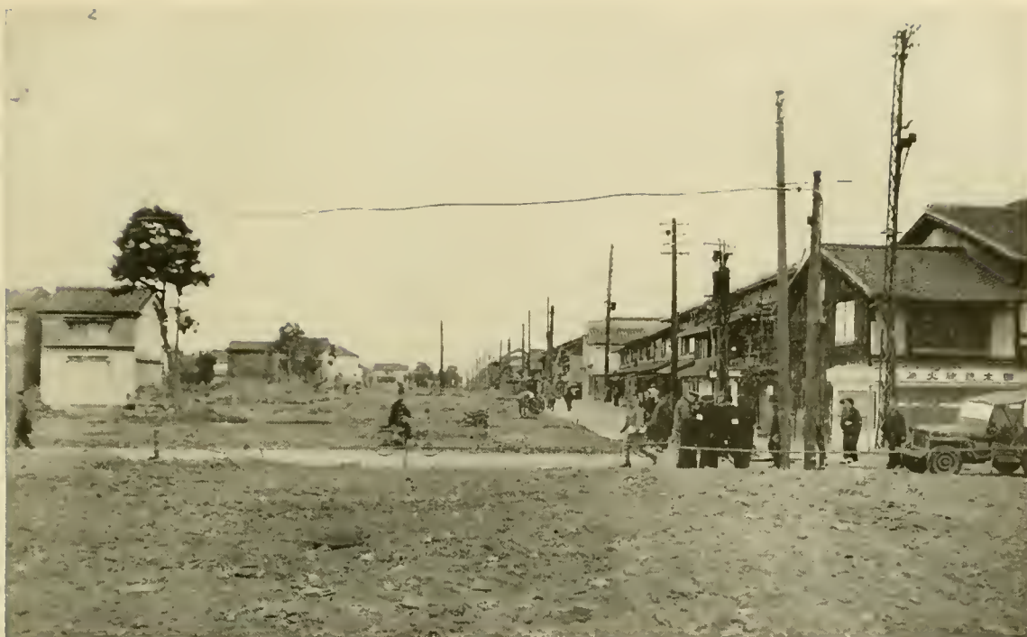
PHOTO 3.—Major cross-town firebreak in Kyoto. All structures have been removed except neighborhood warehouses, such as that on extreme left, which are relatively fire-resistant.
