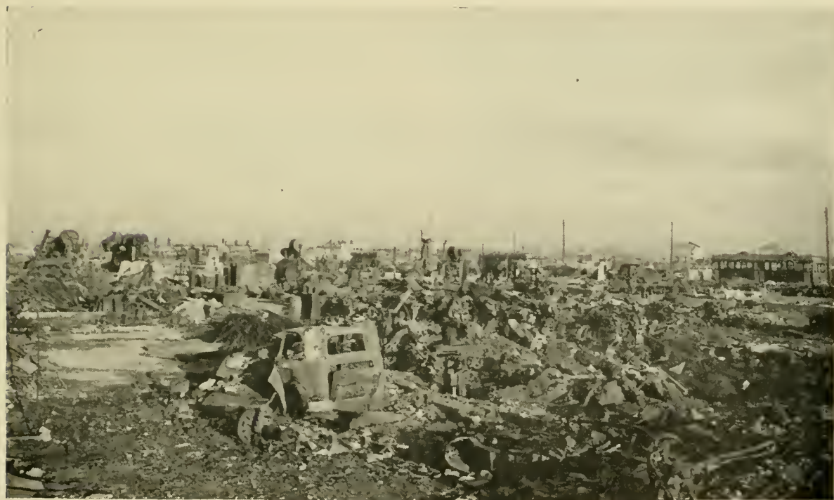
PHOTO 17.—Streetcars dispersed along an Osaka thoroughfare. Dispersal aimed at minimizing losses in terminal fires proved ineffective in districts where conflagrations developed. Remains of three modern high-capacity streetcars may be seen along the street behind this burned-out factory.
