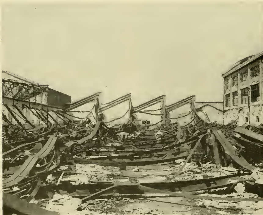
PHOTO 33.—Another type of repair problem. Collapsing roof structures in larger buildings not only caused heavy damage to equipment but delayed salvage of equipment.
