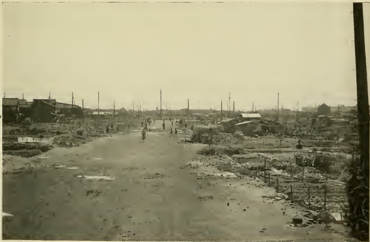
PHOTO 5.—The most ambitious firebreak in Osaka. An extremely wide clearance designed to prevent firespread in the congested northwest industrial section.
