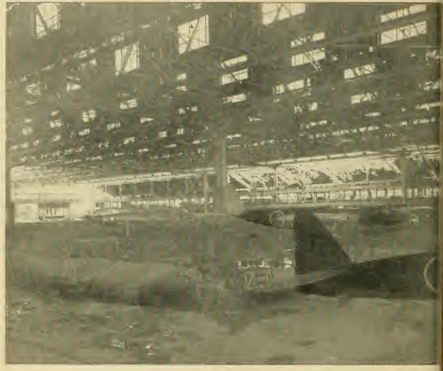
Photo No. 5.—Building 1, final assembly building. View interior, looking northwest, showing assembly lines and slight roof and glass damage.
