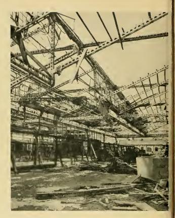
Photo No. 5.—Building 401, final assembly. View west—roof damage over assembly line.
