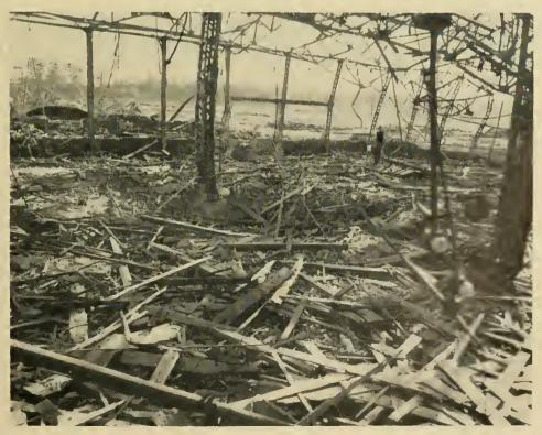
Photo 4.—Building 159, sheet-metal shop. View interior, southwest, showing bomb crater at base of column.
