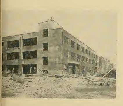
Photo No. 4.—Buildings 701, 704, 716, machine shops and sheet metal works. View north, showing bomb damage of direct hits and near-misses to a steel-reinforced concrete building.
