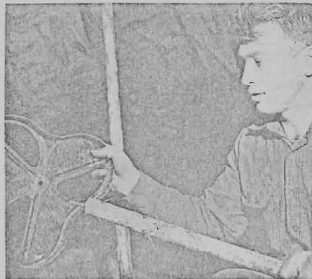
Cloverleaf prevents tearing camouflage netting.
