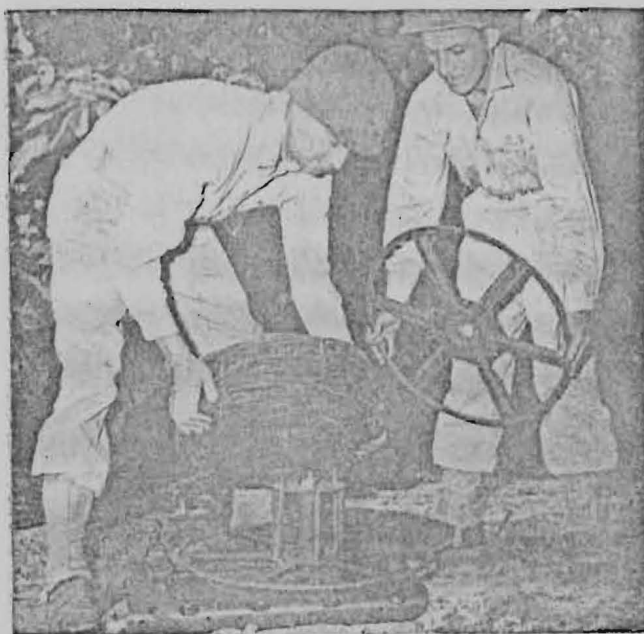
The wire slips onto modified DR-4 Reel.
