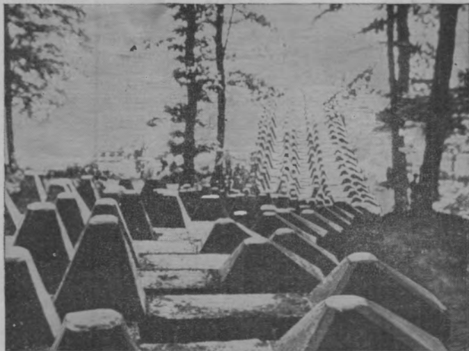
Figure 9. Dragon's teeth, showing four double rows.
