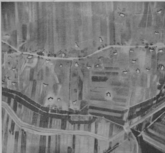
Figure 11. Aerial view of a portion of the West Wall during construction, showing shapes of emplacements.
