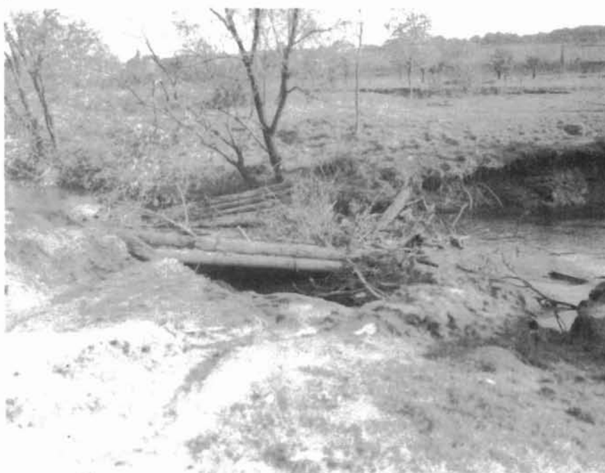
Tank bridge expedient This failed due to boggy-ness of terrain near the river bank
