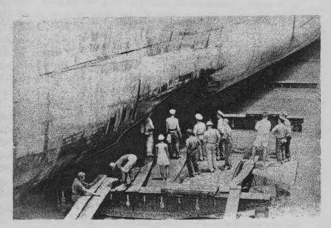
Damage to hull of Marblehead, port side forward, the result of a near hit in Madoera Strait.
