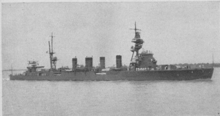
SENDAI 8/37 NOTE CUTTER BOW—JINTSU, NAKA HAVE HOOKED BOW
