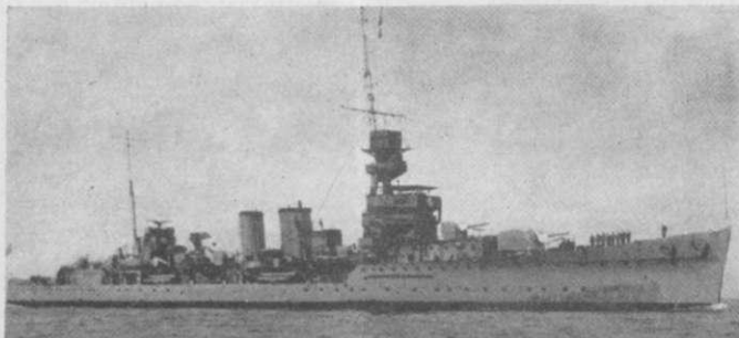
DIOMEDE—note gun-house to No. 1 6-inch gun; only ship so fitted.
