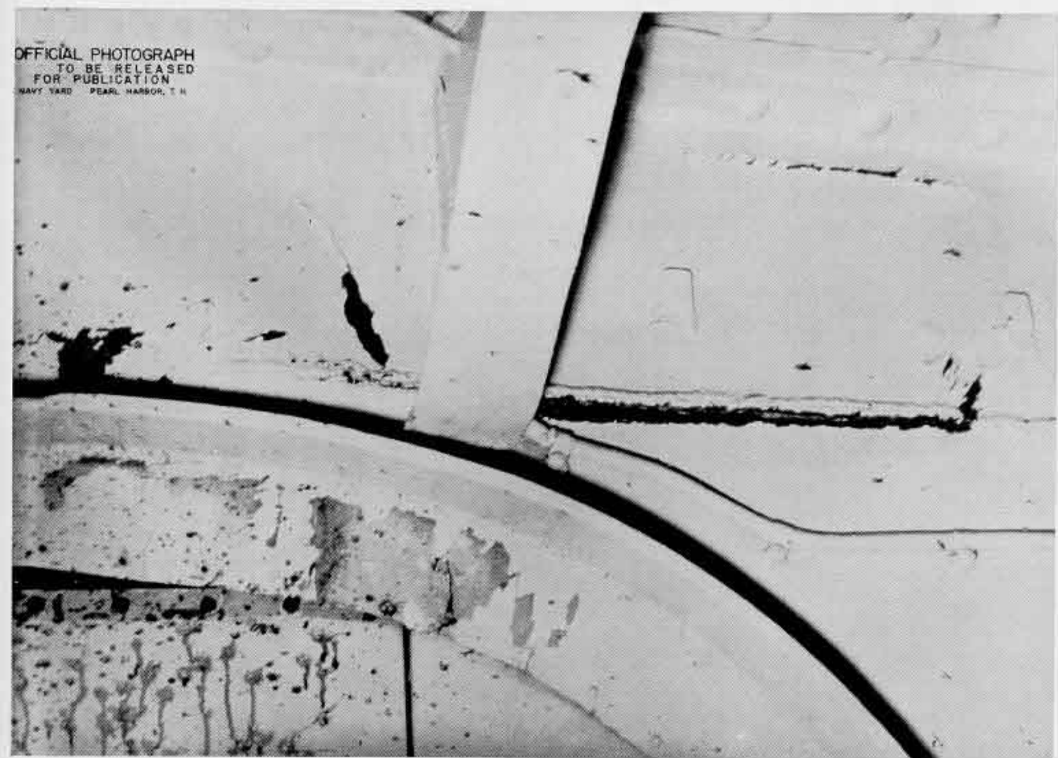
Photo 22: Web FR 109, underneath 2nd deck, bracket to starboard shell, looking forward. Note rupture at weld.
