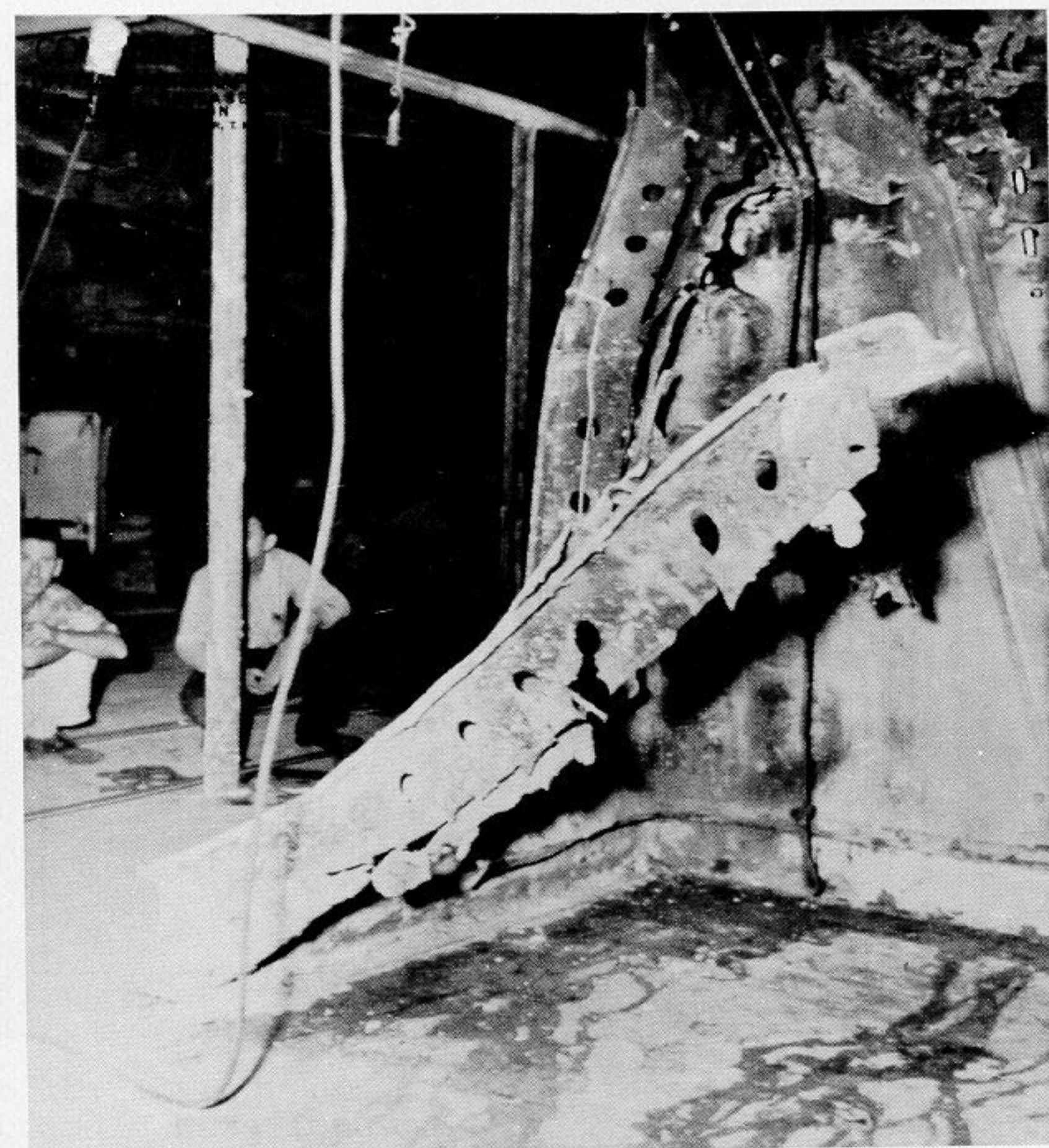
Photo 16: Damage to Bulkhead 106, between 4th and 3rd decks, looking aft.
