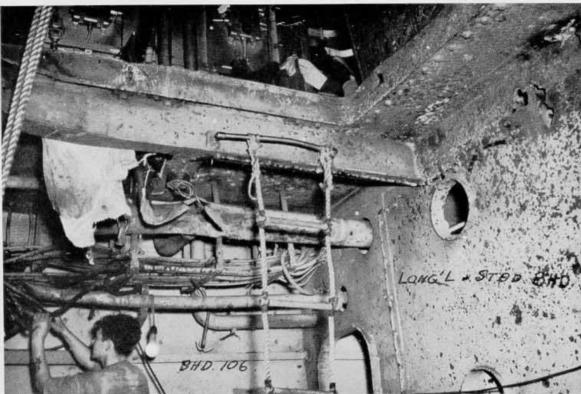
Photo 30: Fragment damage, starboard longitudinal bulkhead, second deck, FRS 106-109, looking forward.
