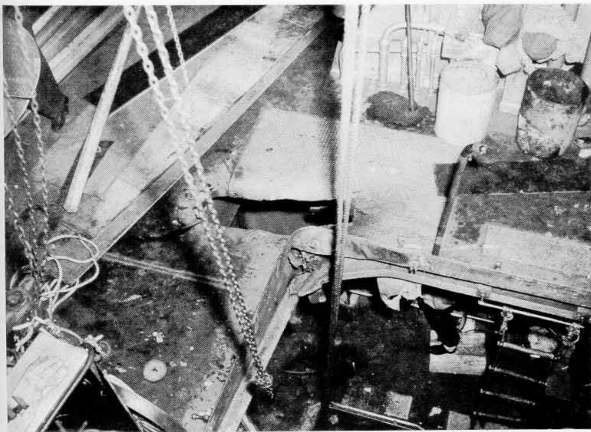
Photo 8: Bomb Hole, Main Deck, FR 107 1/2 looking down.
