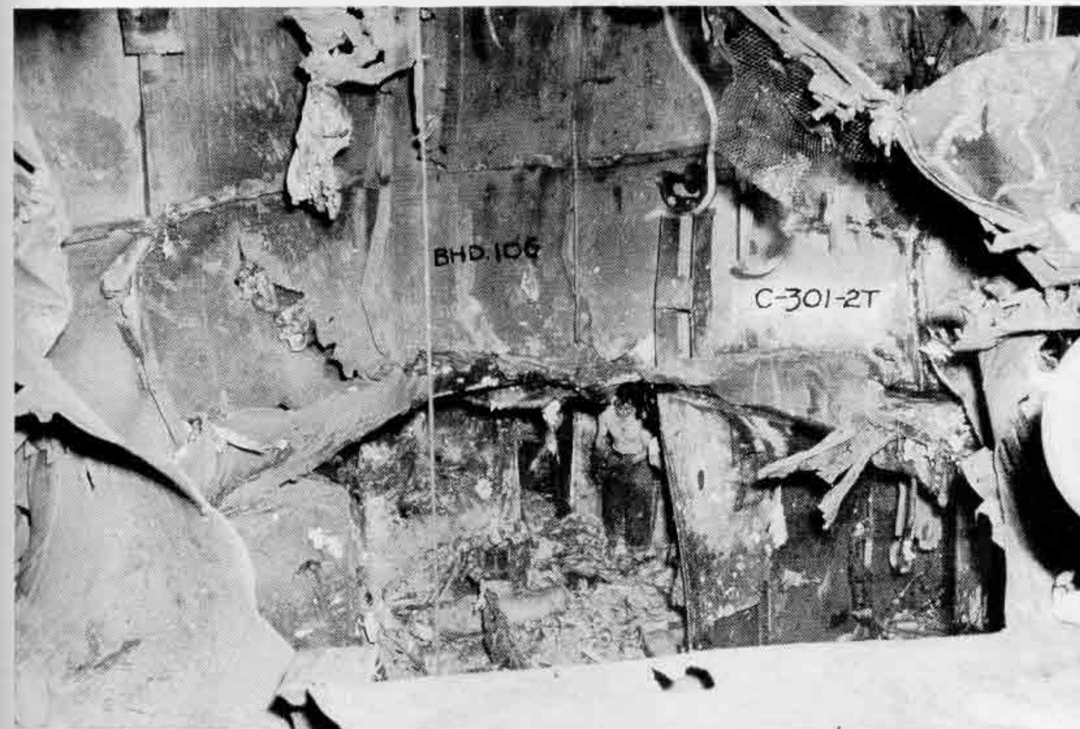
Photo 12: Blast Hole in Third Deck. Some wreckage cleared away. Looking forward and down.
