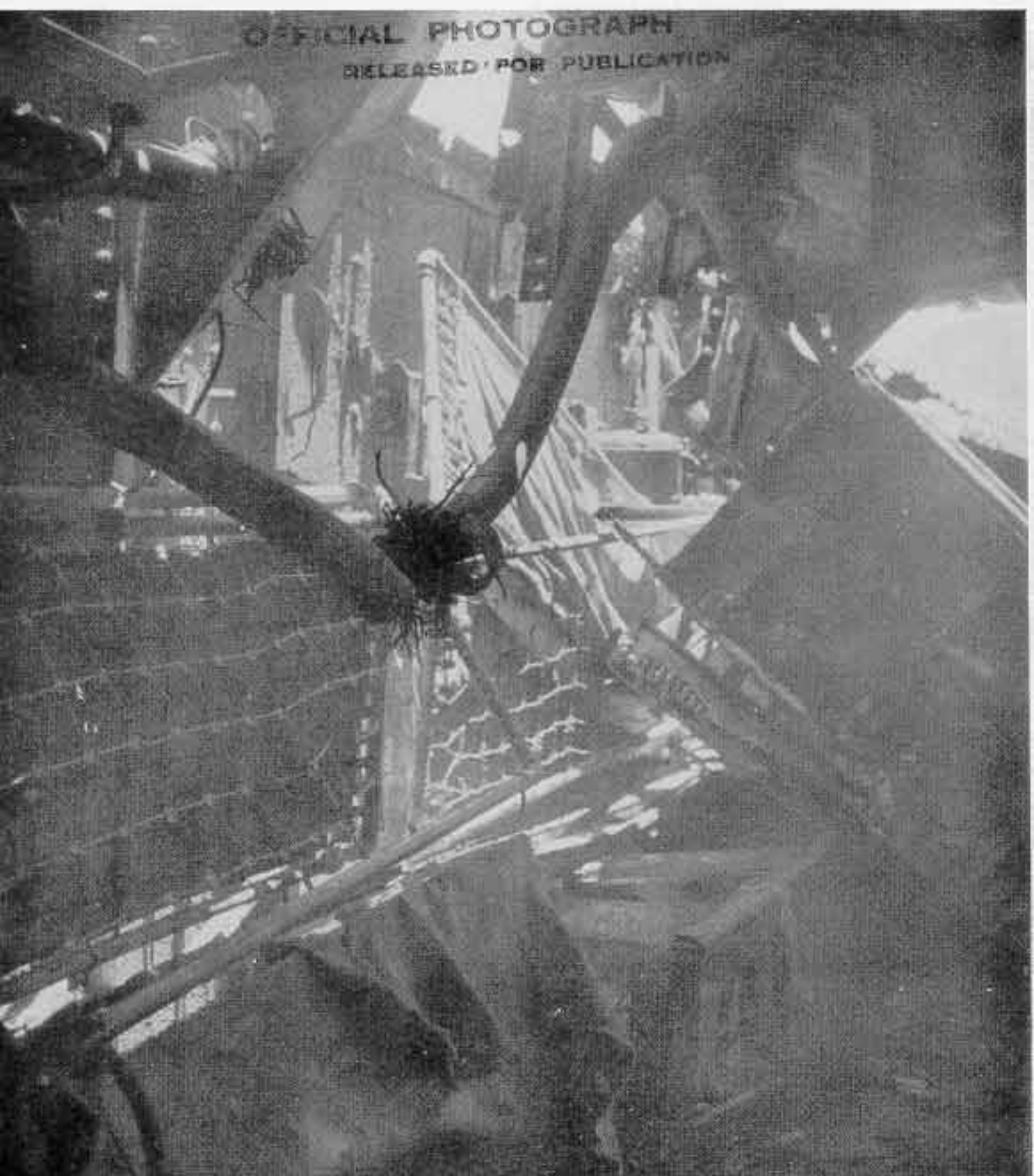
Photo 4: C.P.O. quarters D-304 port side.
