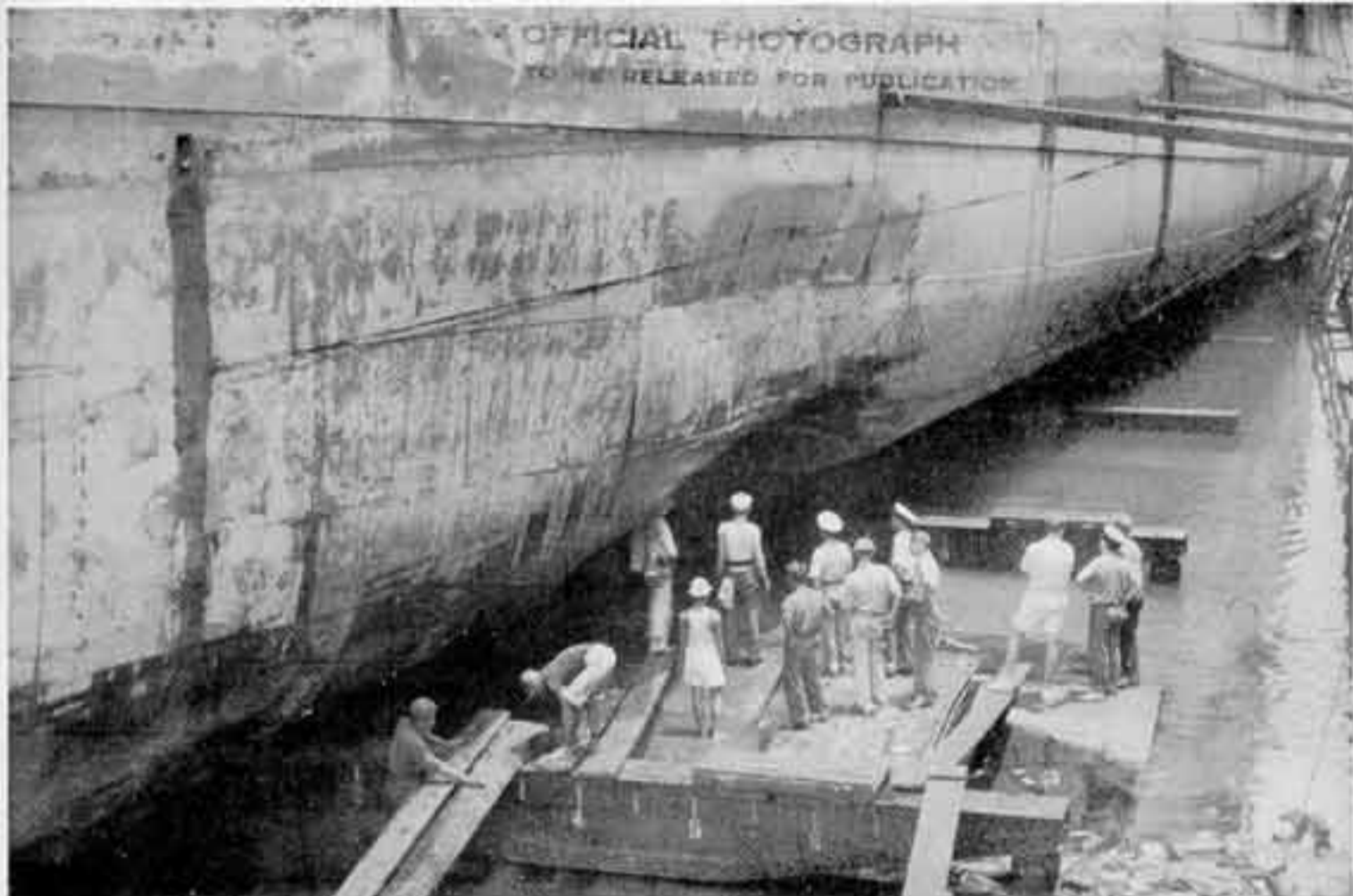
Photo 17: Near miss showing bulge port side.
