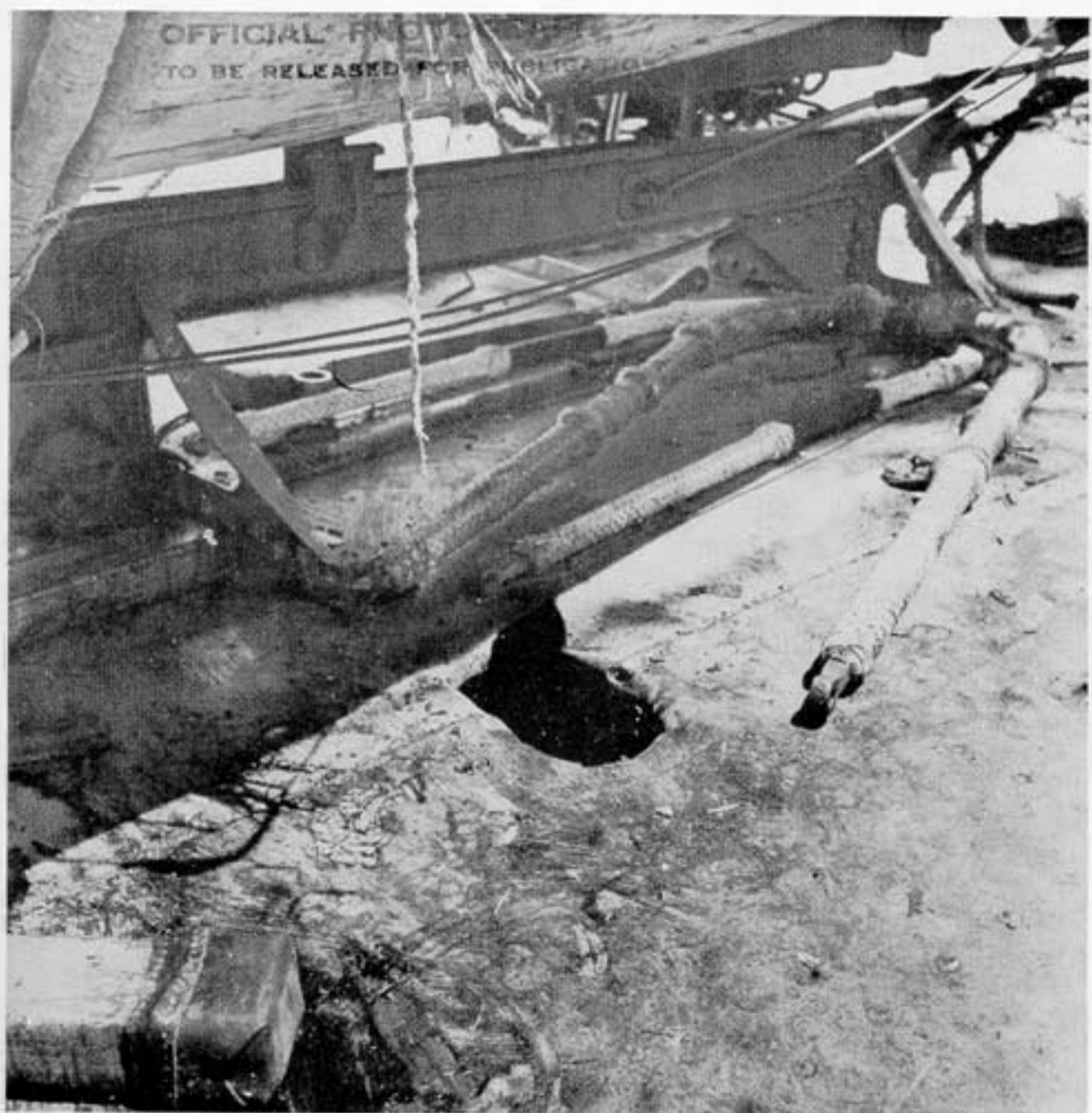
Photo 12: Bomb hole upper deck under motor launch.
