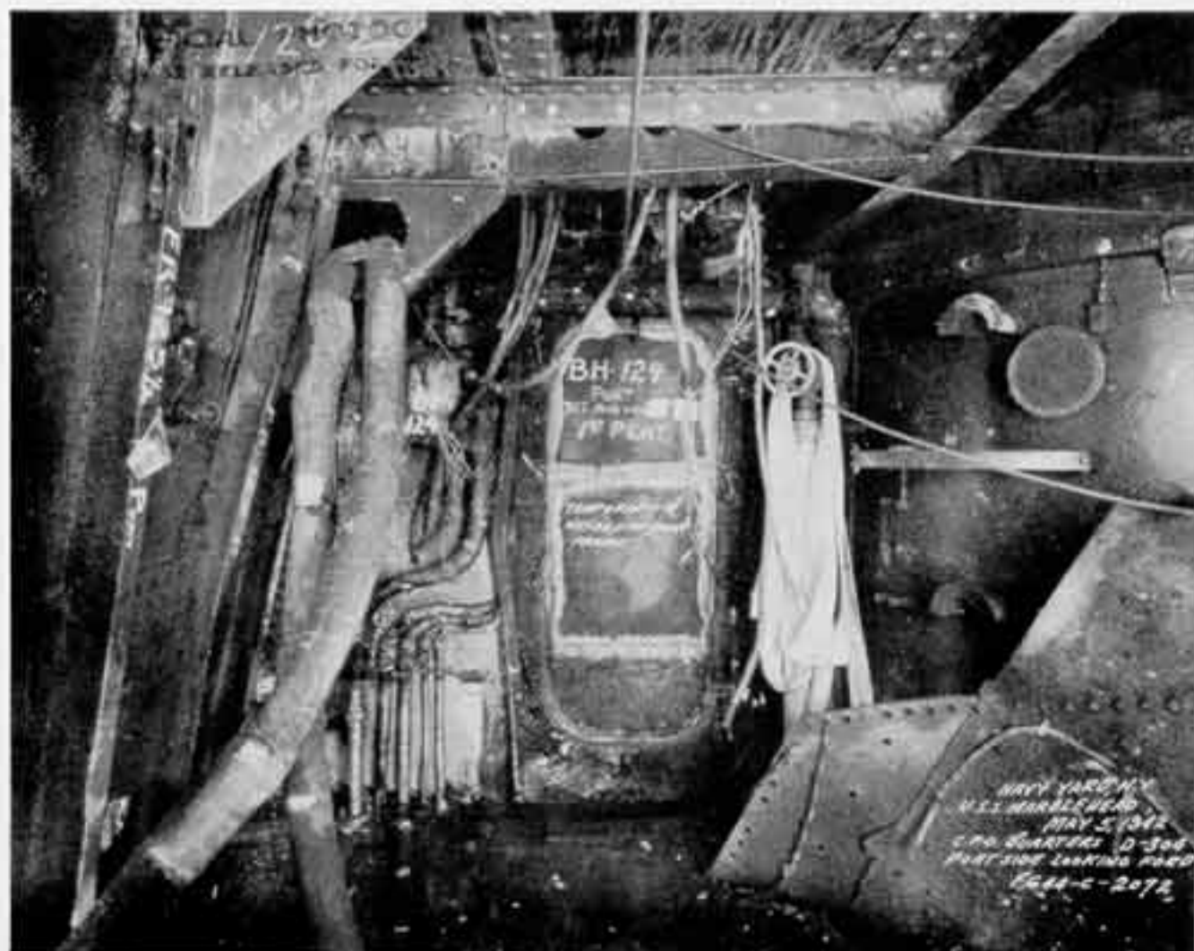
Photo 6: C.P.O. quarters D-304 port side looking forward.
