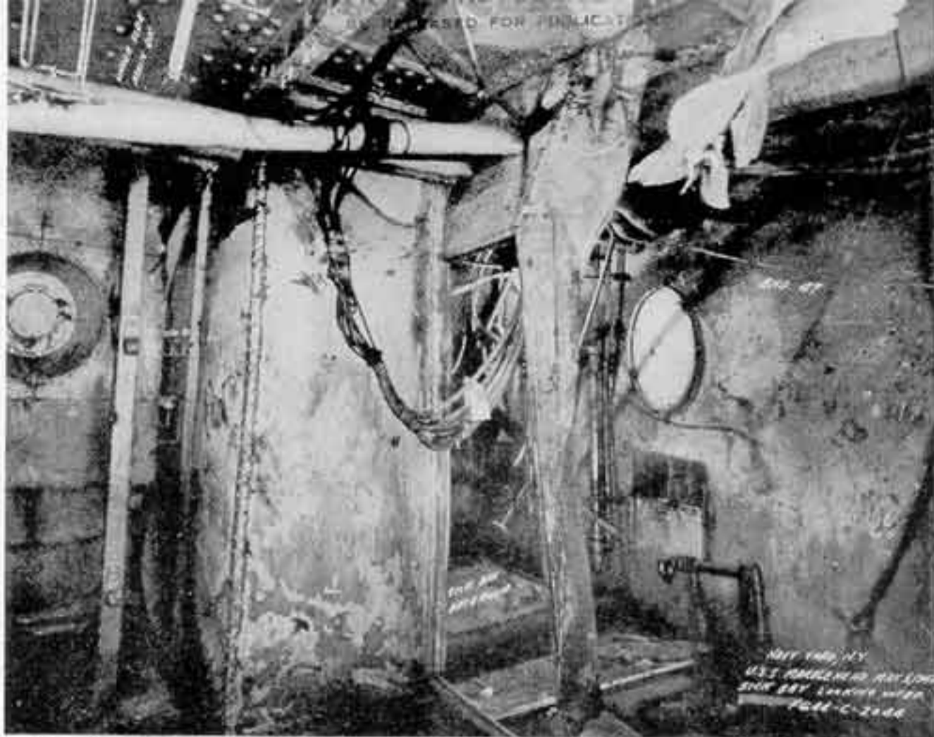
Photo 15: Sick bay first platform deck looking outboard.
