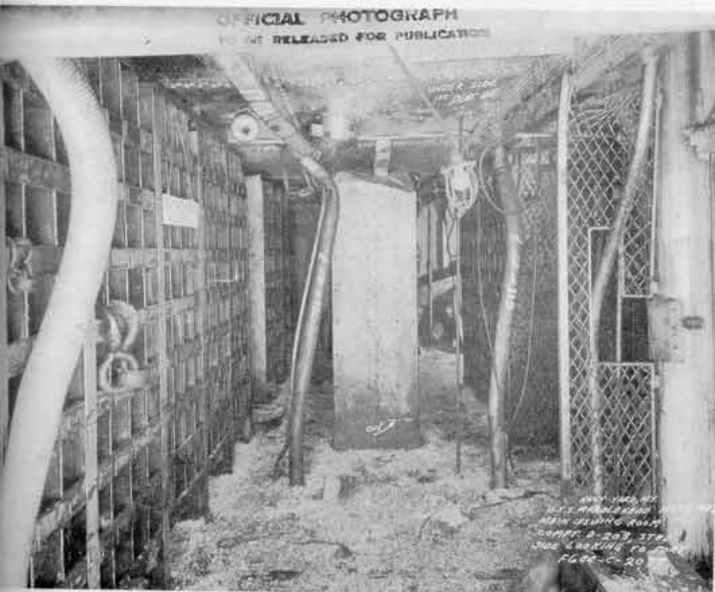
Photo 10: Compartment D-203, starboard, looking to port.
