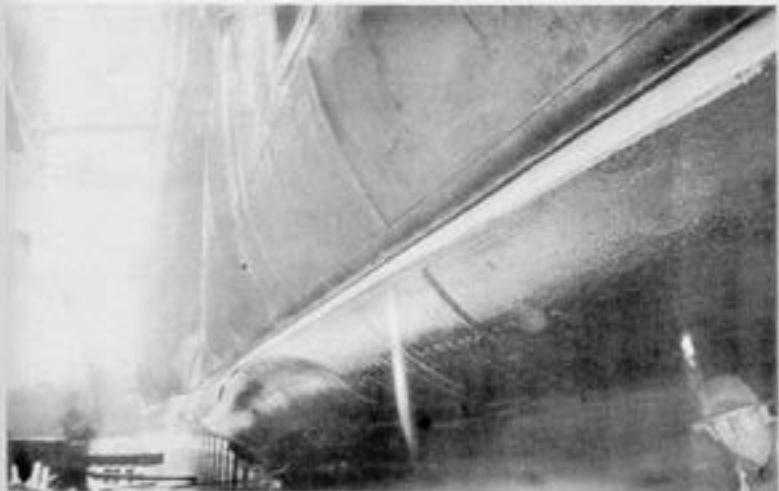
Photo No. 7: View looking forward along port bilge keel. Note how the bottom plating inboard of the bilge keel was blown down by the explosion.
