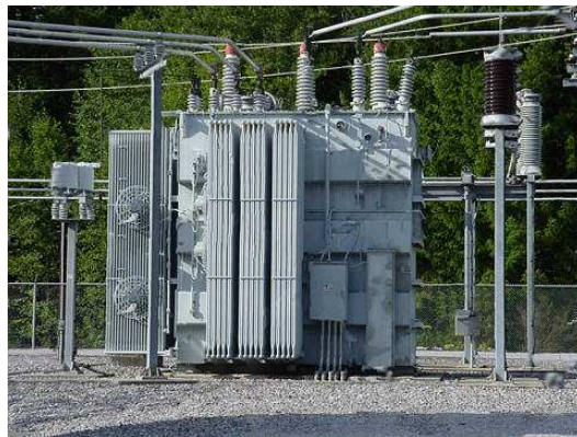
Figure 9.20: Substation transformer.
