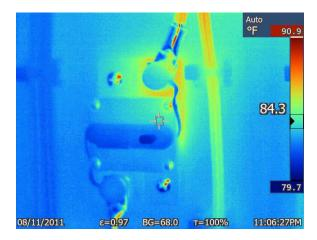
The yellow "glow" radiating outward on the surface of the circuit breaker from the upper terminal reveals heat generated at the interface between the wire's metal terminating lug and the bolt where that lug attaches to the circuit breaker. The dull yellow coloring of the wires themselves similarly reveals the heating effect of electric current passing through.
