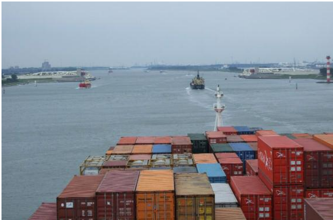
The MONTE SARMIENTO seen approaching the "Maeslant Flood barrier" outward bound from Rotterdam Photo : Peter Elsinga ©
