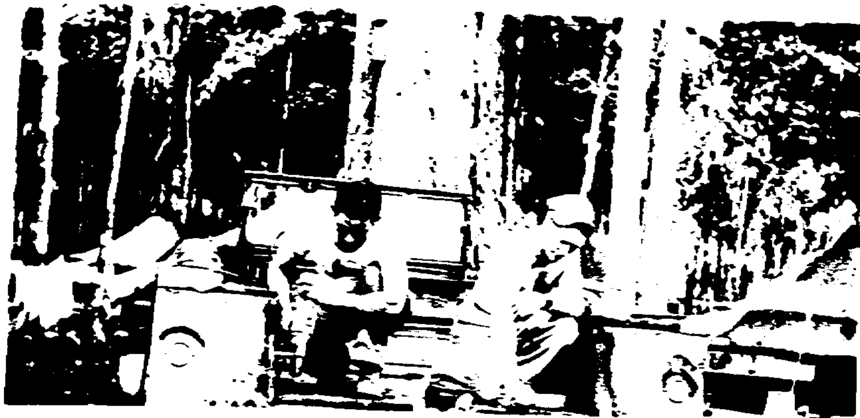
Auto Mechanics Putting in New Bed in Truck 1024th Signal Co Sv Gp, 6th Service Group (Air) Photo taken by 6th Sv Gp (Air) Photo Section 30 December 1944.
